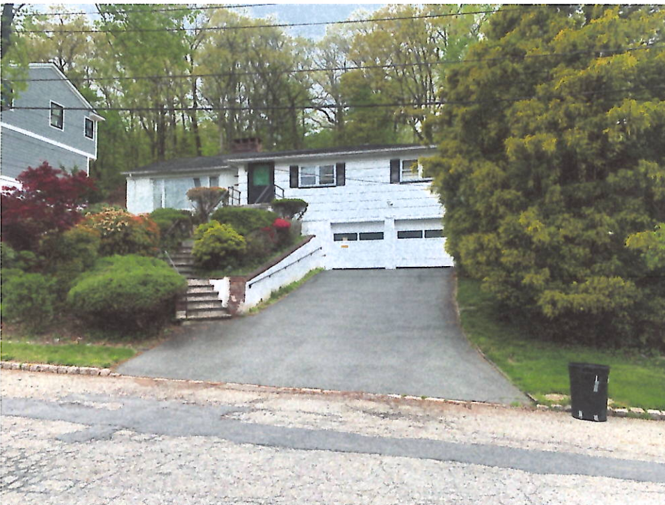
Photo 4 House immediately to the North on Cleveland. Note railing on wall coming down from the garage.
