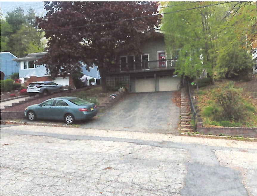
Photo 2. House immediately to the south on Cleveland. Note parking area in the street Right of Way and stairs with a railing on the right side.
