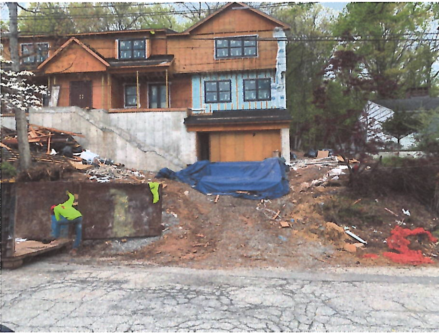
Photo 1 The front of the subject property under construction with a conforming addition. The existing driveway going straight up from the street has an average slope of 23%.
