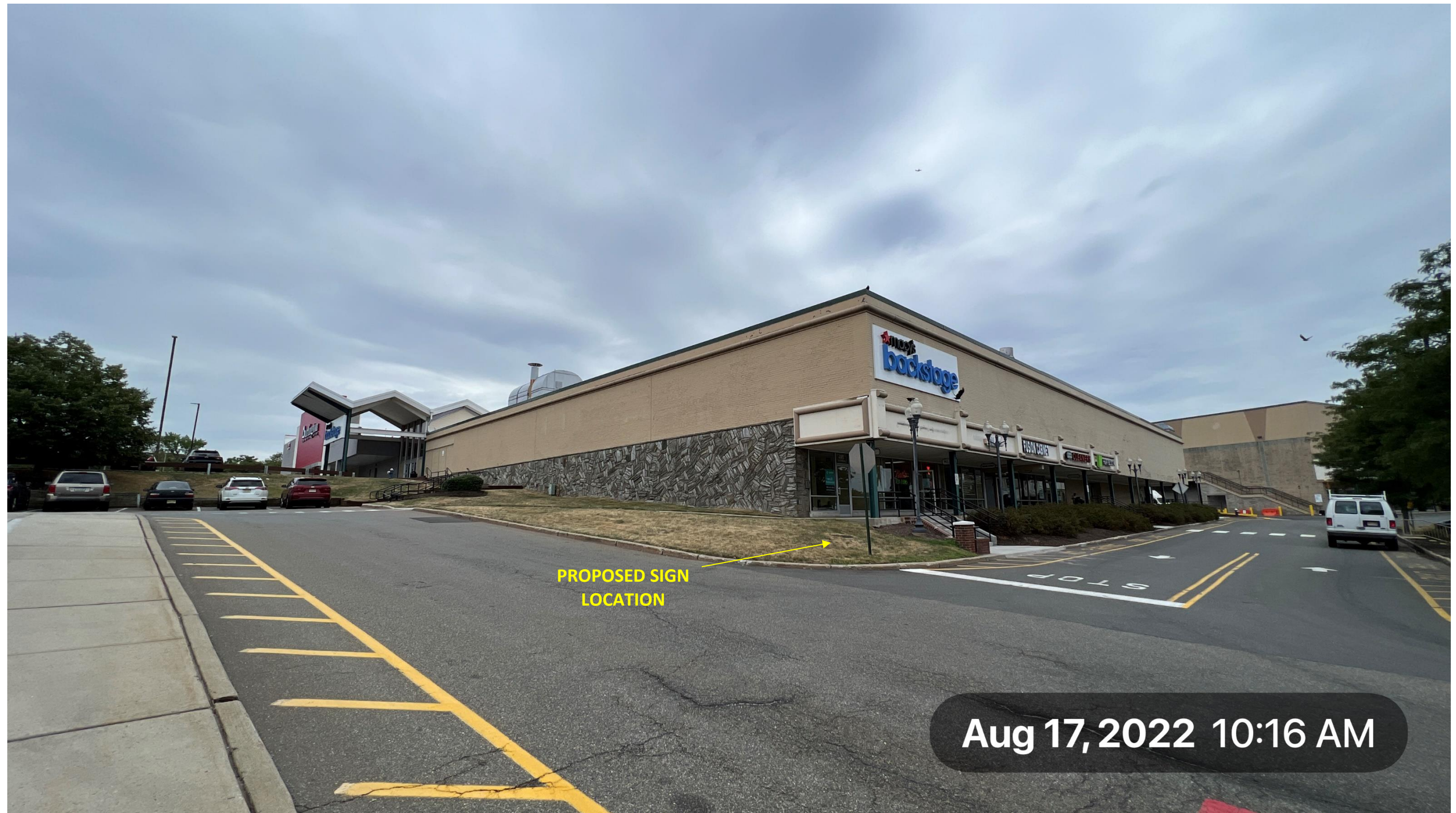
GROUND VIEW OF SUBJECT SITE LOOKING SOUTHEAST (TAKEN BY JOHN MCDONOUGH ASSOCIATES ON AUGUST 17, 2022)
