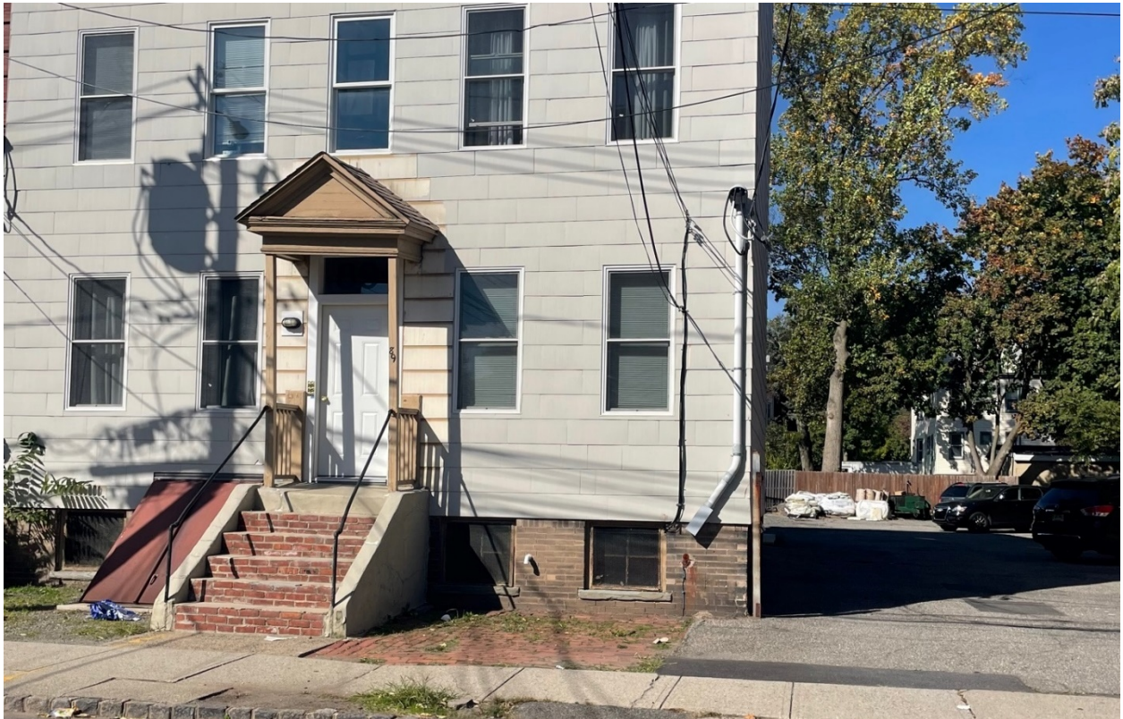
Front of existing building and driveway
