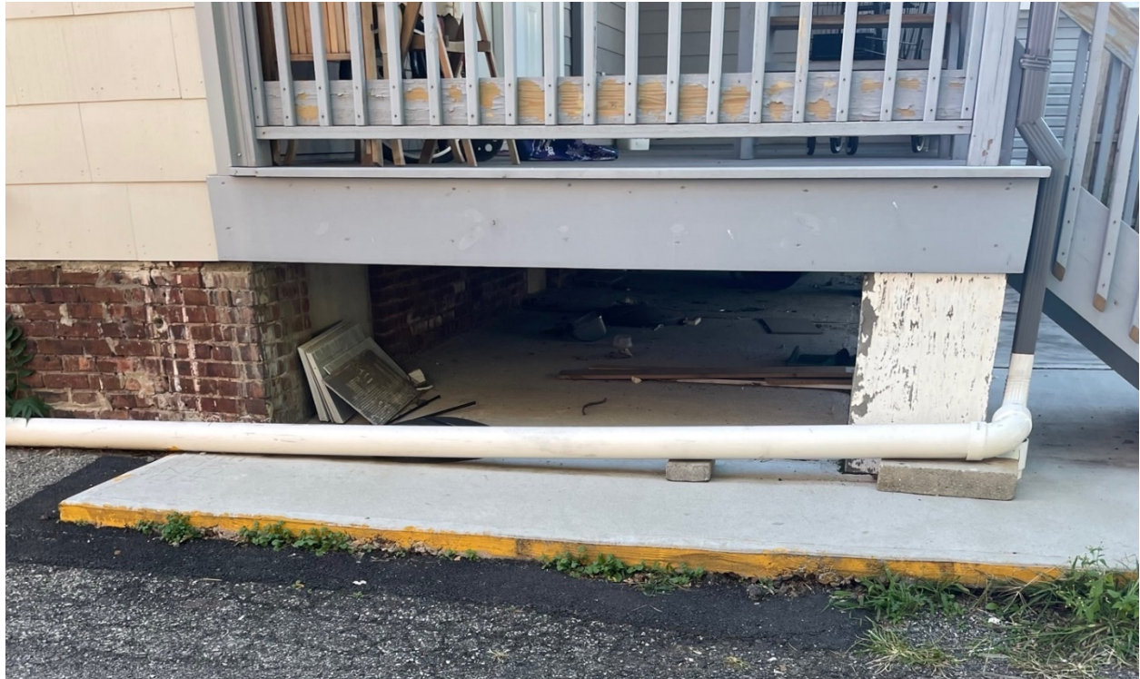
Rear views of property (top) and rear porch of existing building (bottom)
