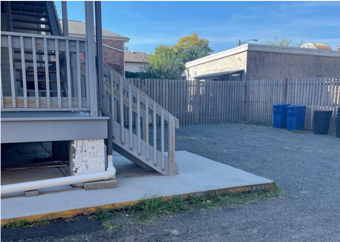
Rear stairs and yard of existing building
