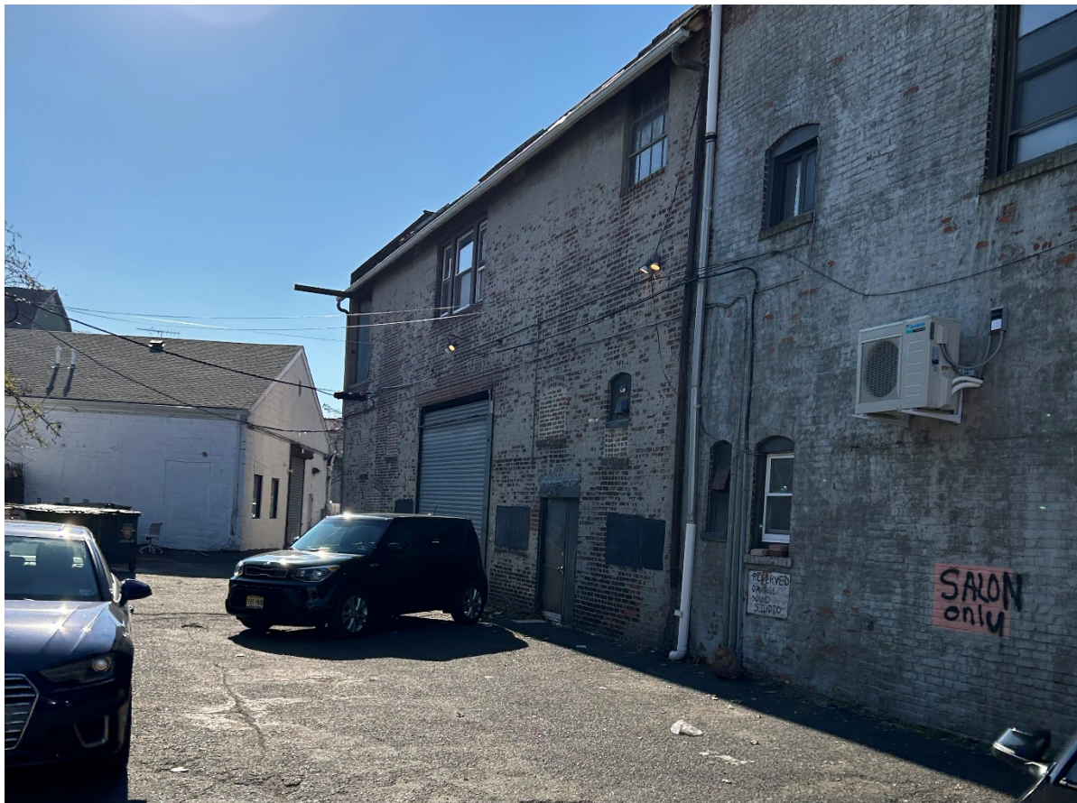
Existing parking area and east side of building
