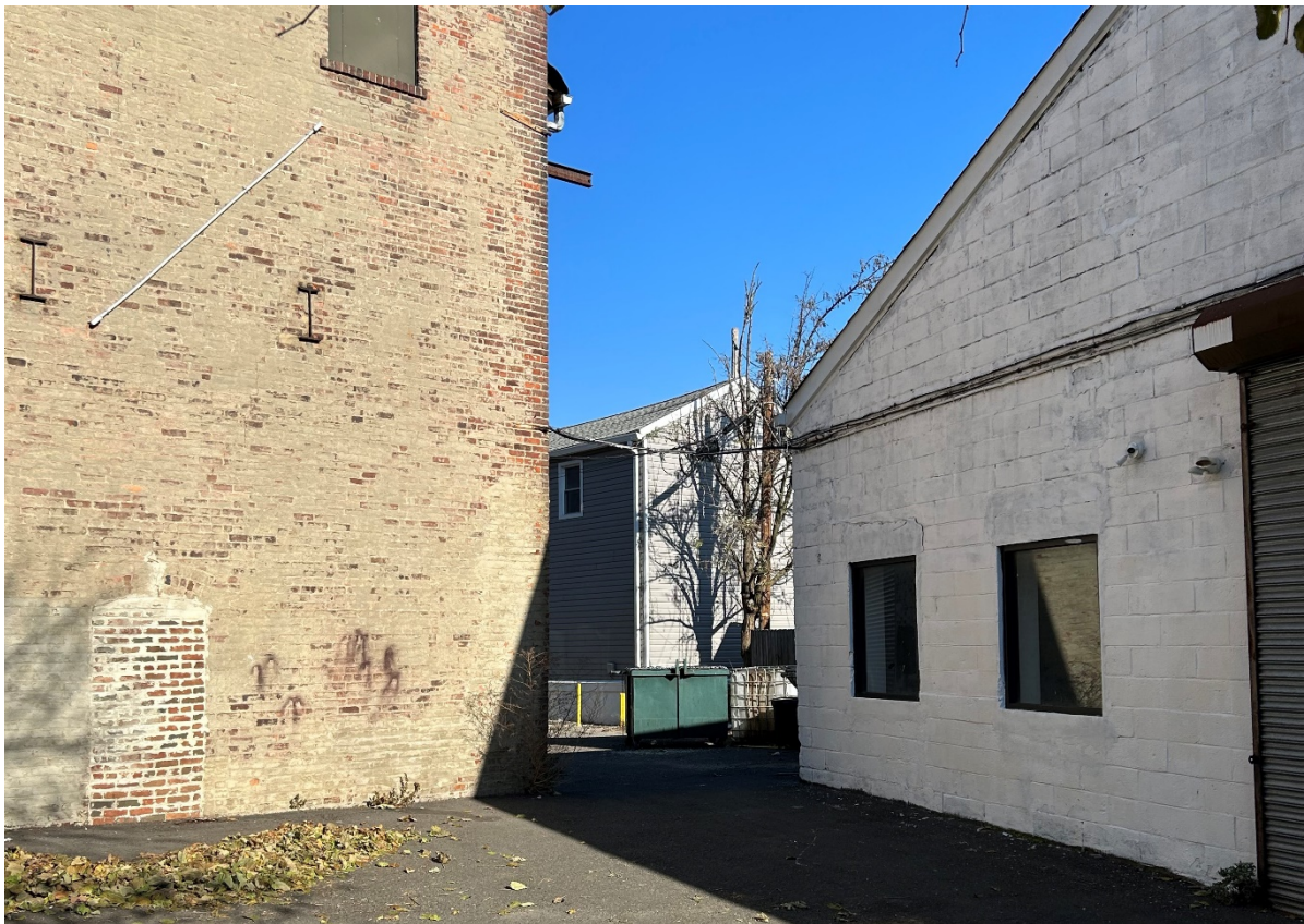
Rear of building (top) and access to Lot 5, including building on Lot 5 on right (bottom)
