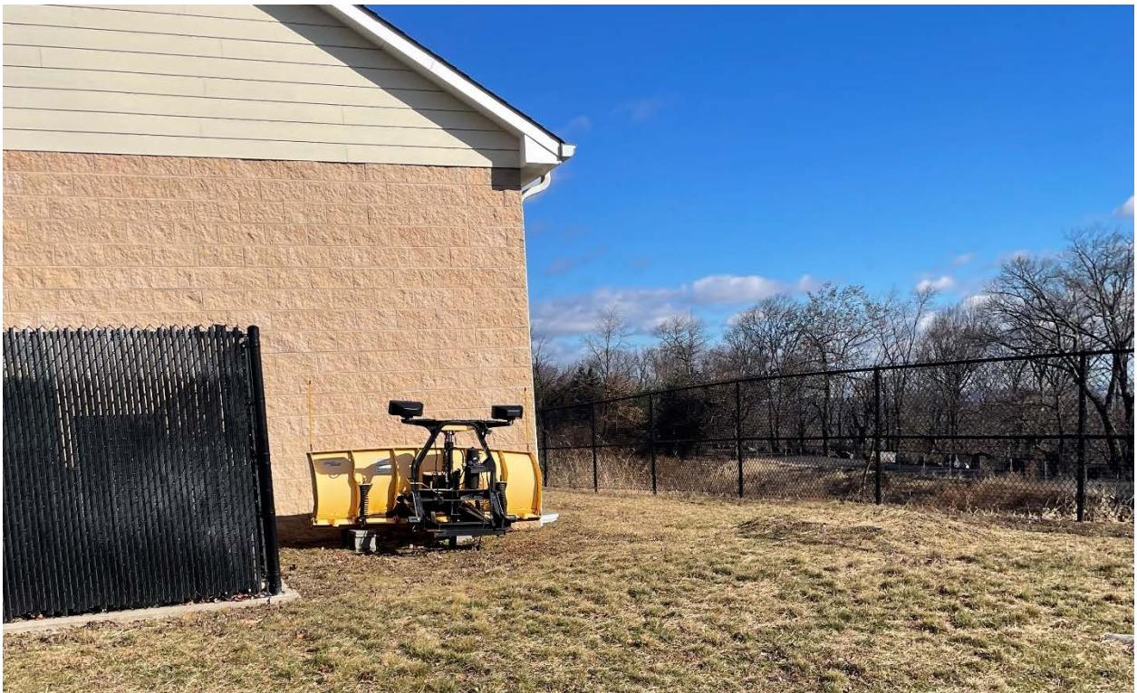
Rear of existing building
