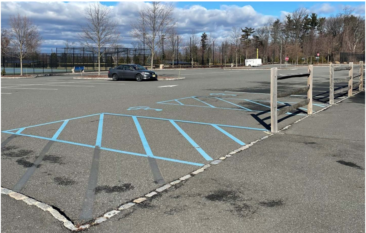
Edge of closest parking area to proposed expanded building
