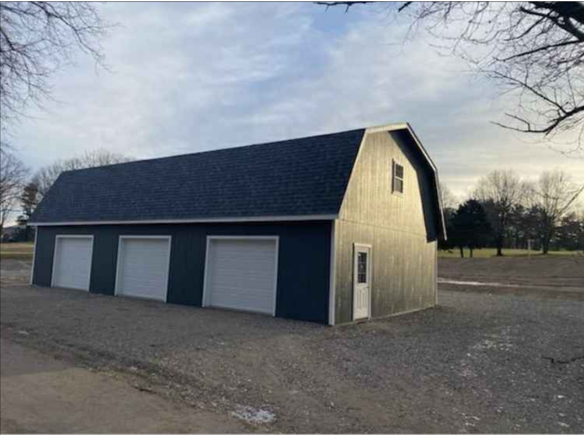
MAINTENANCE STORAGE SHED PHOTO Photo from Hendrick,s Field Golf Course
