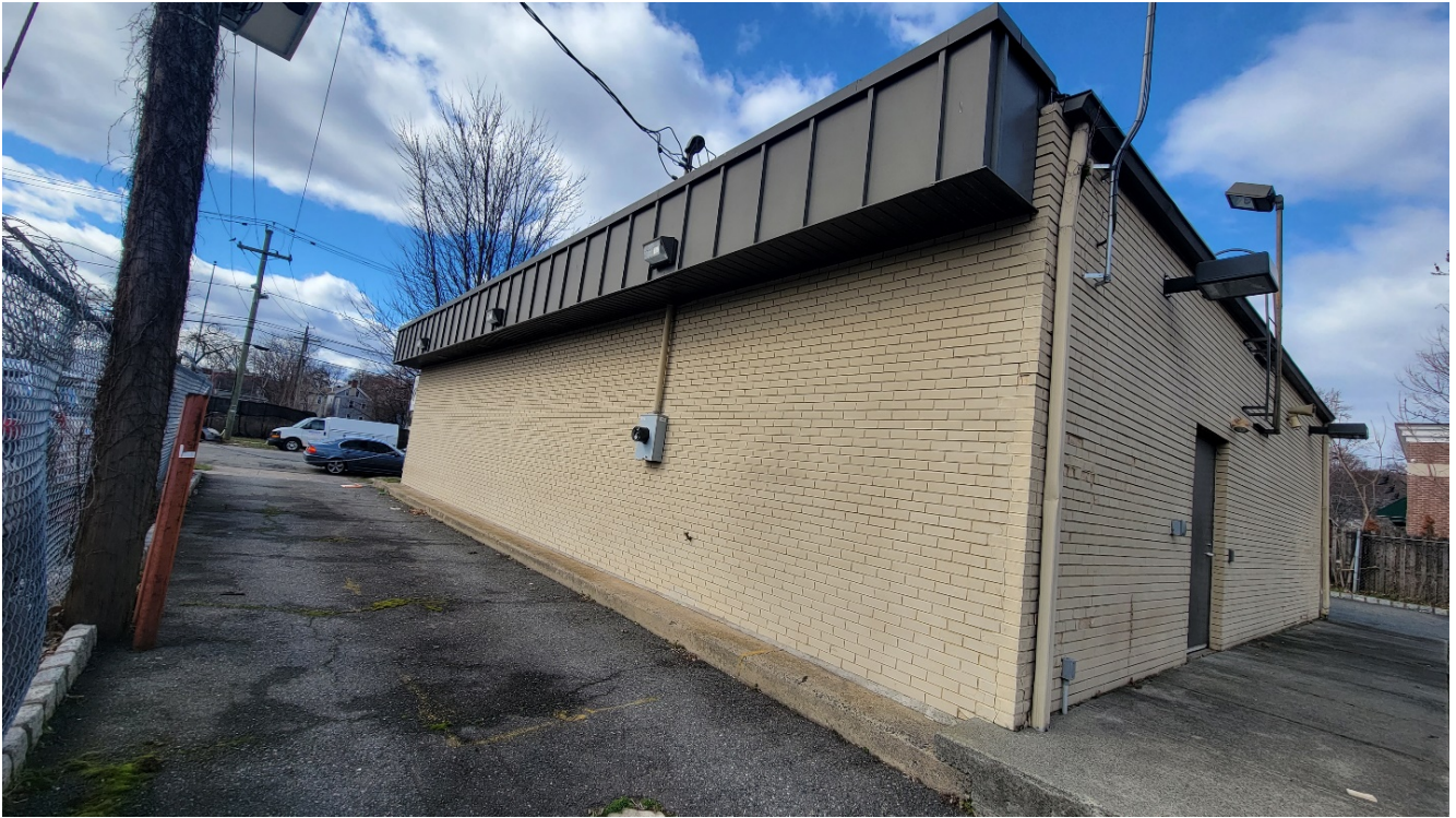
East side of building
