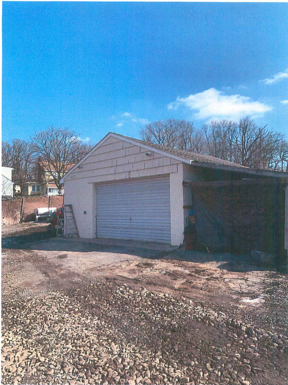
Existing Garage in Rear Fenced Area
