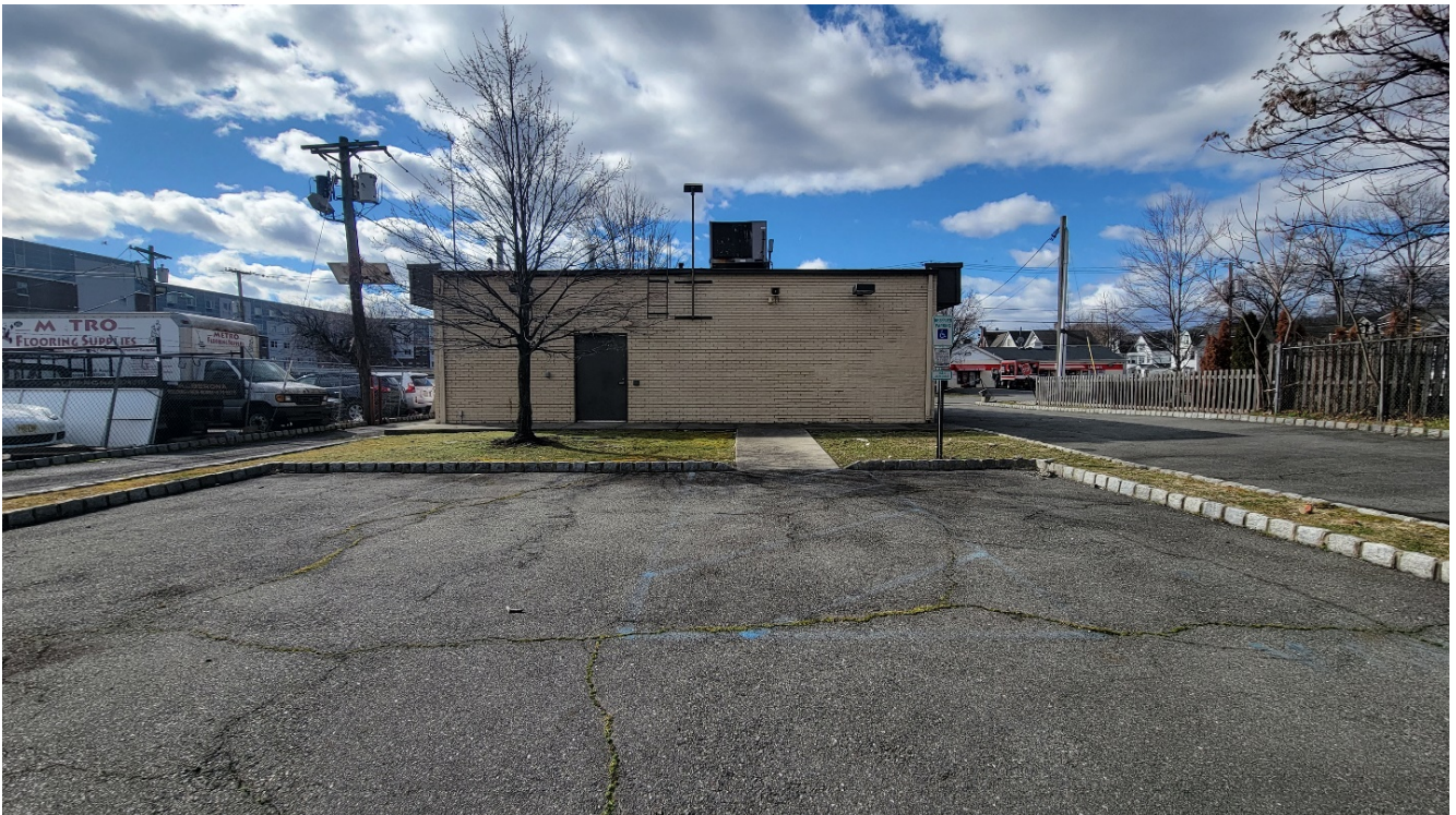
Rear of building and parking lot
