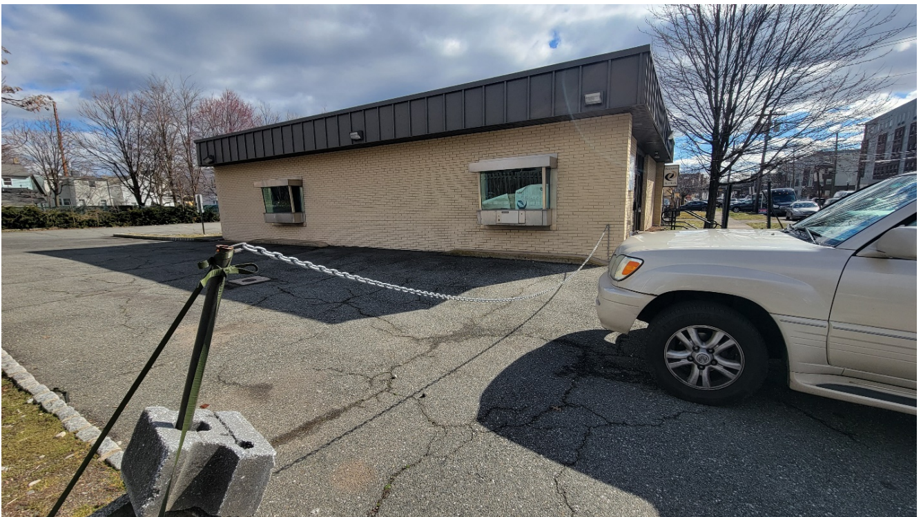
West side of building, including existing drive-up windows
