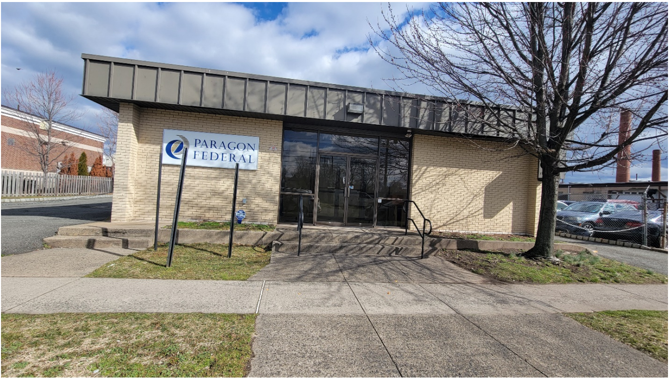
Front view of building
