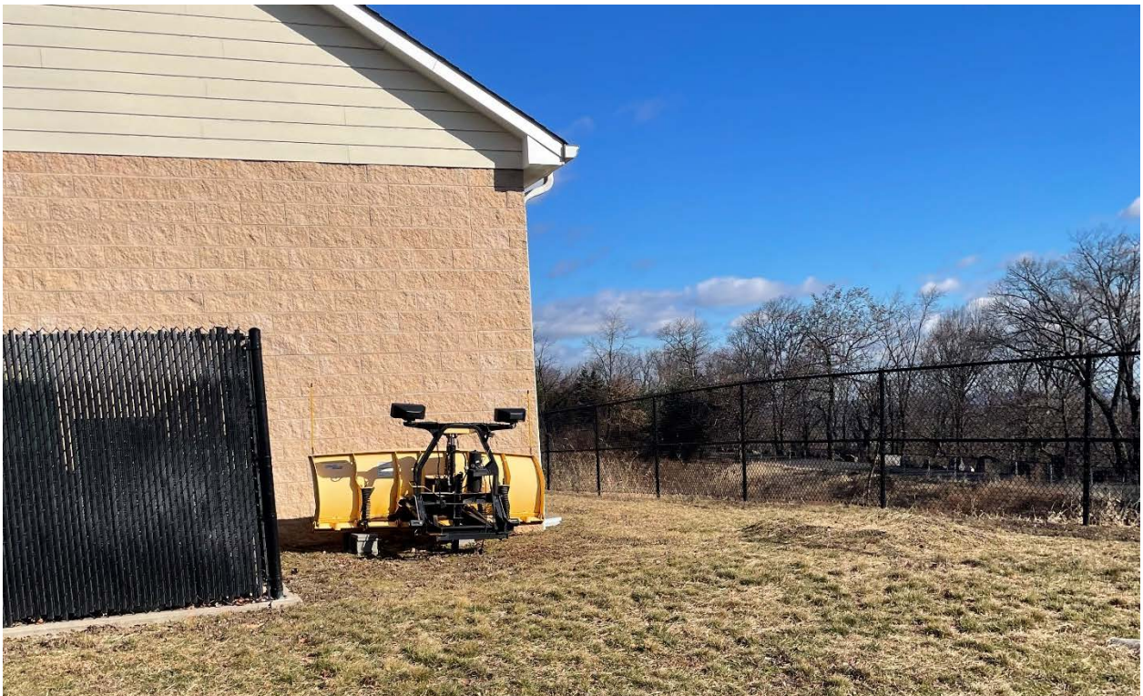
Rear of existing building
