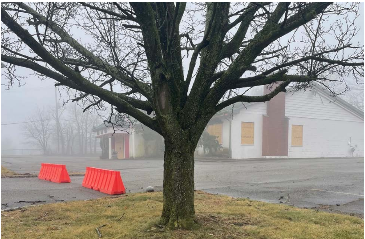
Front views of property
