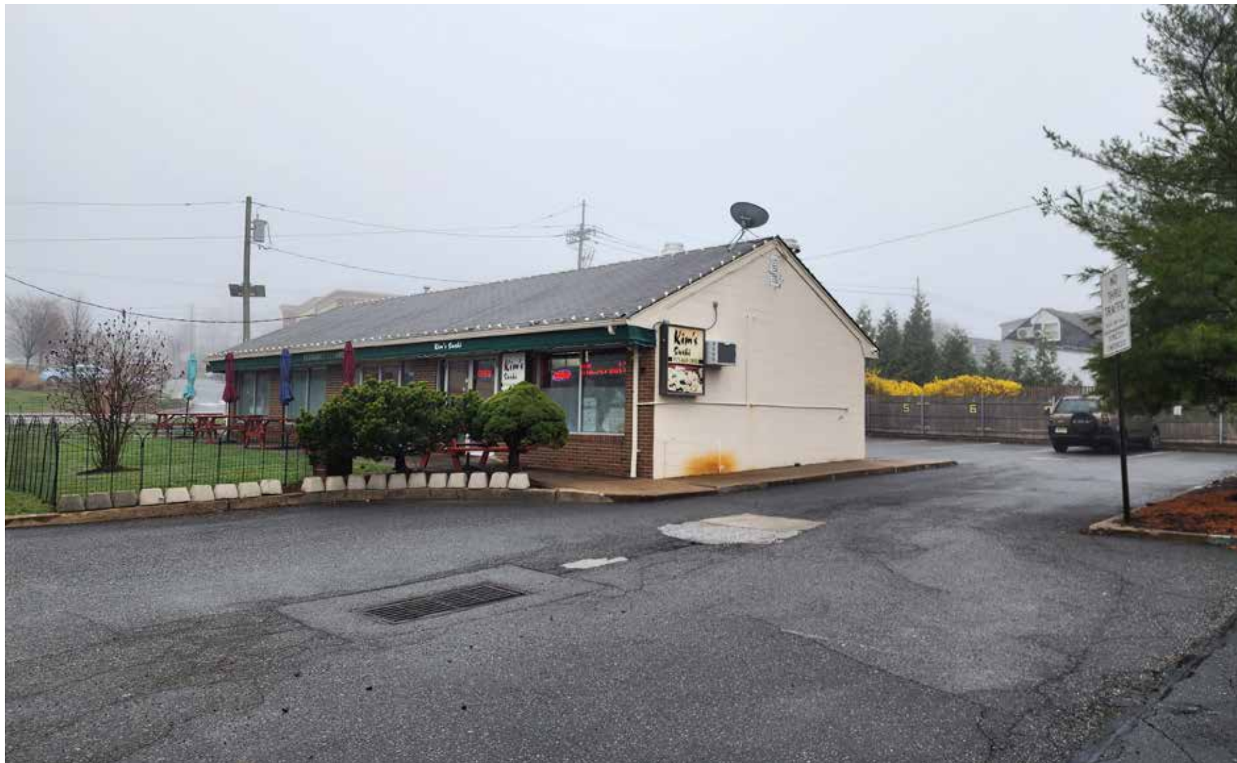
Photo 2: 456 Eagle Rock Avenue
