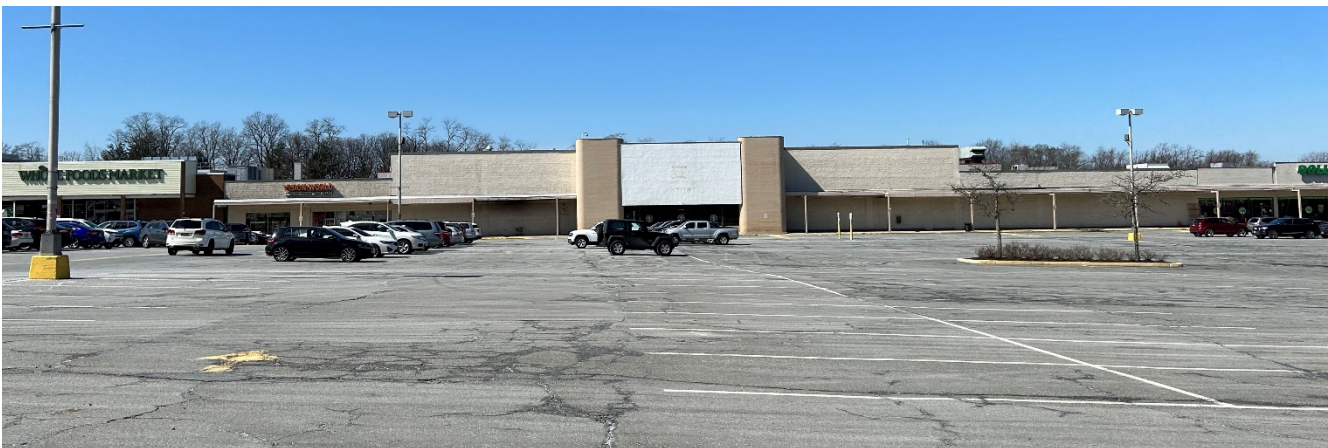
Views of front of former K-Mart building where Target is proposed
