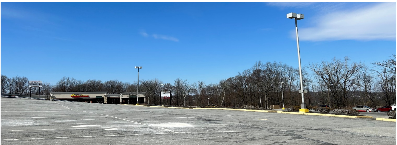
Northern portion of main building and location of proposed Building A
