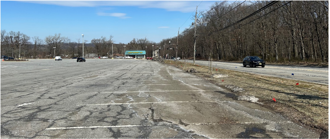
Portion of site where Building C is proposed
