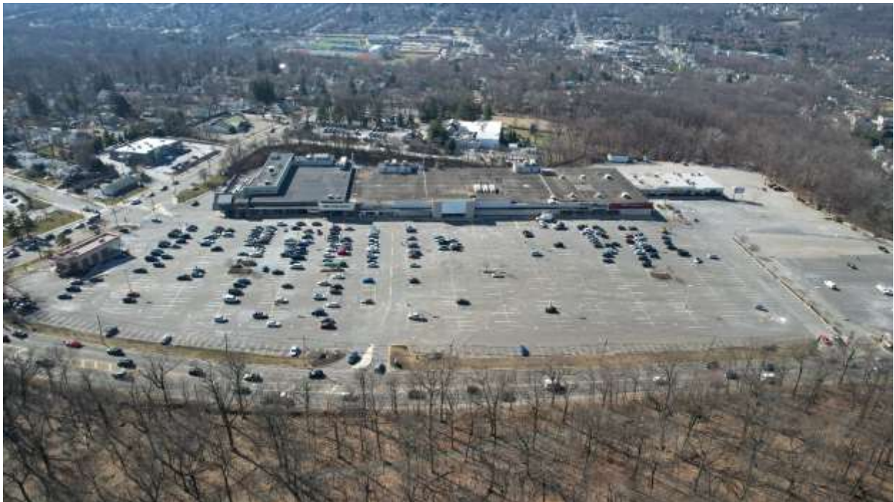
Figure 12 – Aerial drone view of subject site looking west (taken by John McDonough Associates on March 20, 2023)
