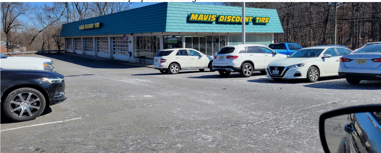
Existing Mavis building, to be renovated with garages removed
