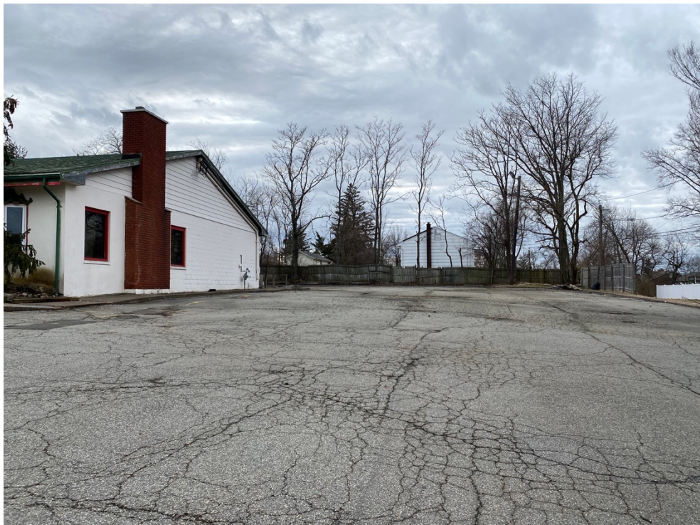
Photo 4: The southerly portion of the project site consists of an impervious surface parking area, which previously consumed 88.3% of the site). The proposed lot coverage conditions would be a decrease, amounting to approximately 71.2%.
