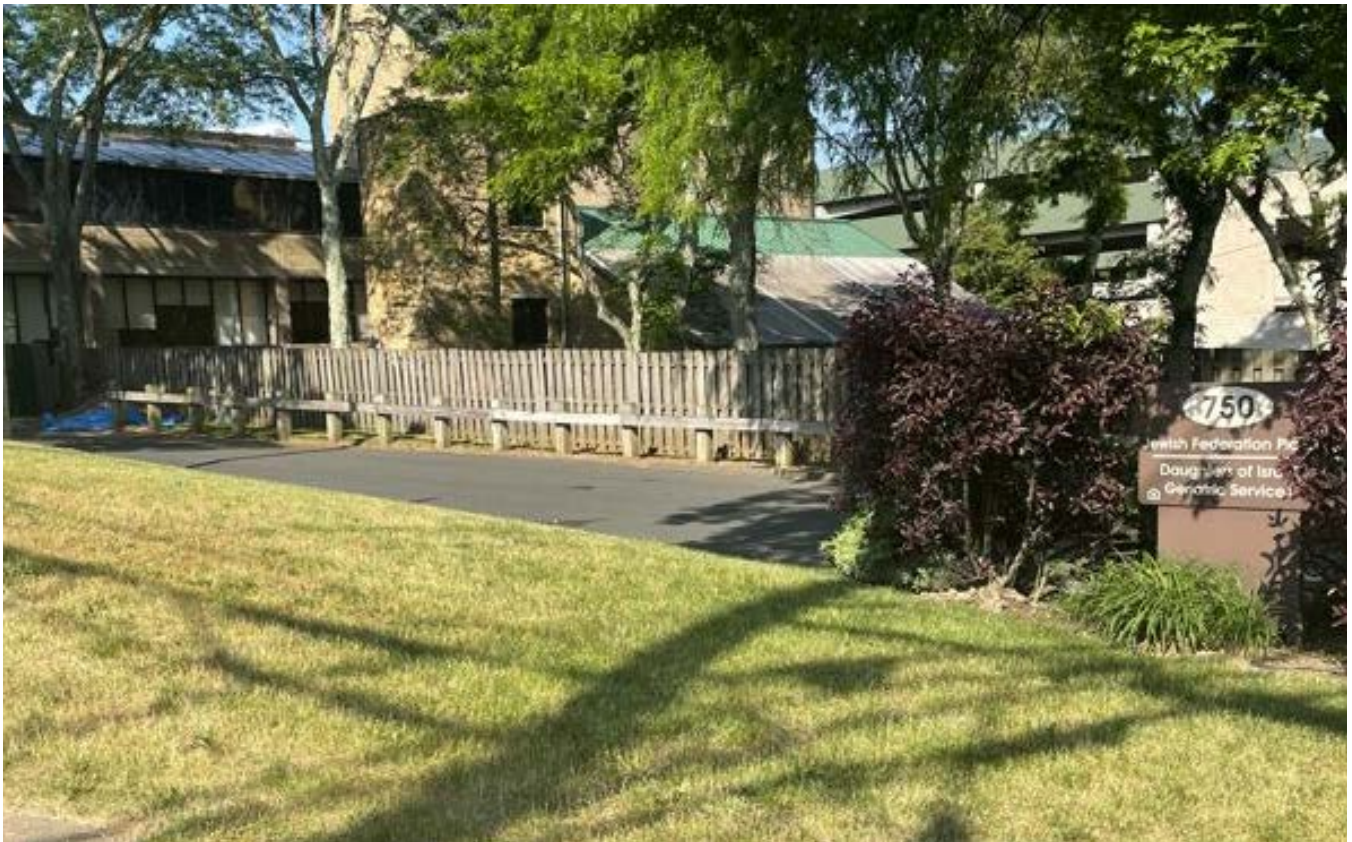
Looking west and southwest to driveway and existing sign
