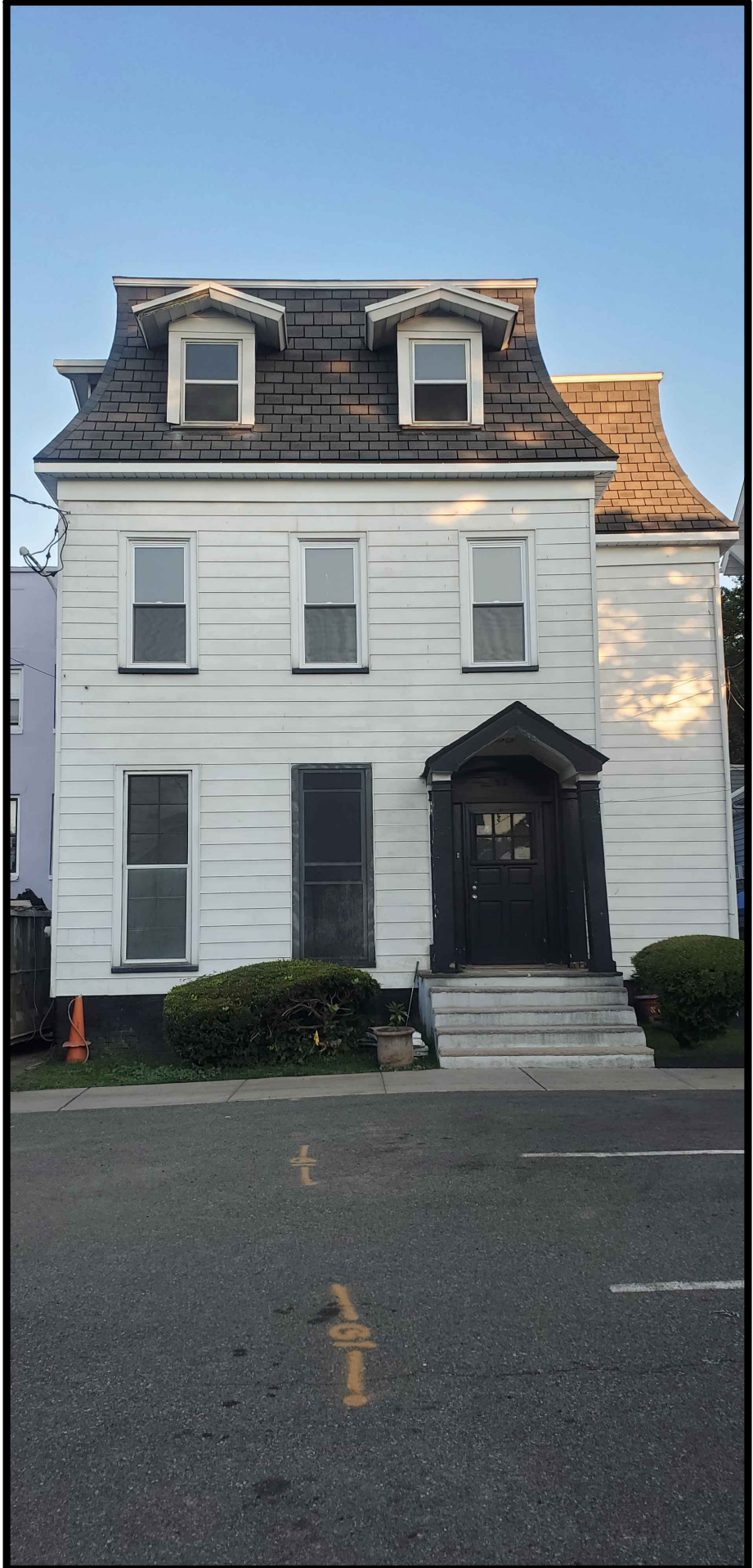
CLOSER VIEW OF FRONT OF BLDG.
