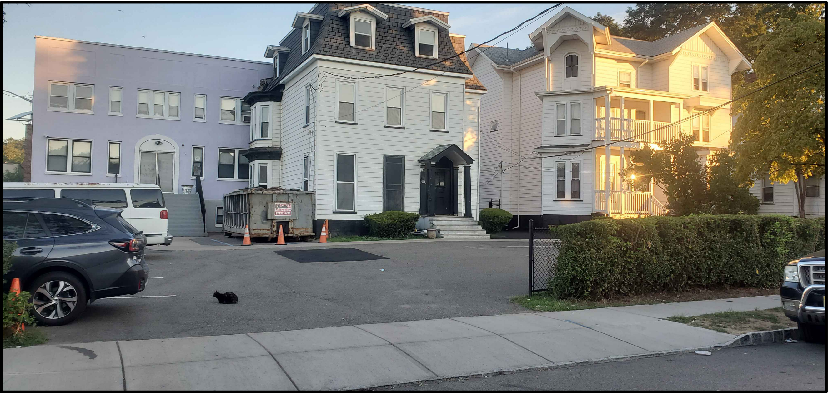
VIEW OF SITE FROM TOMPKINS STREET
