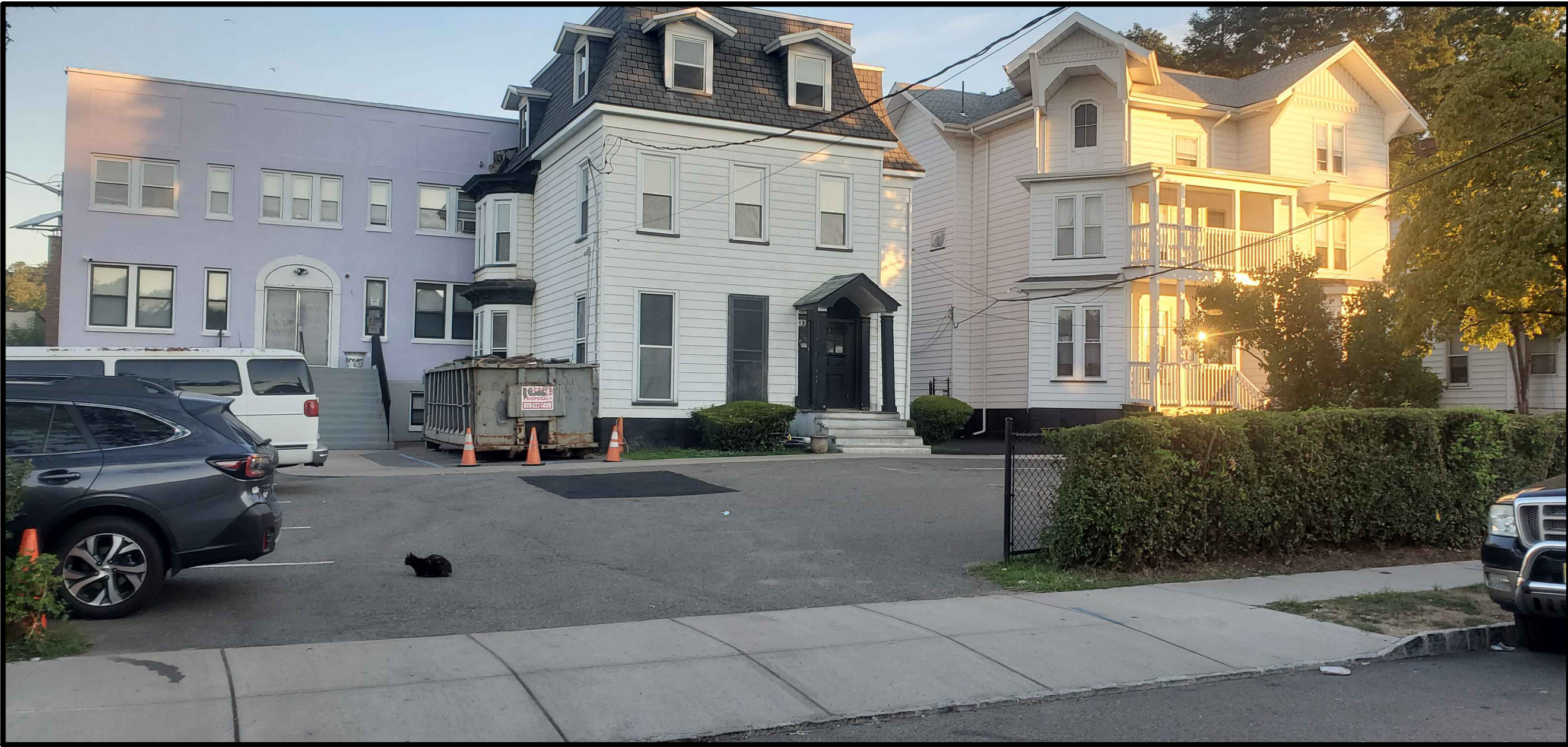
VIEW OF SITE FROM TOMPKINS STREET
