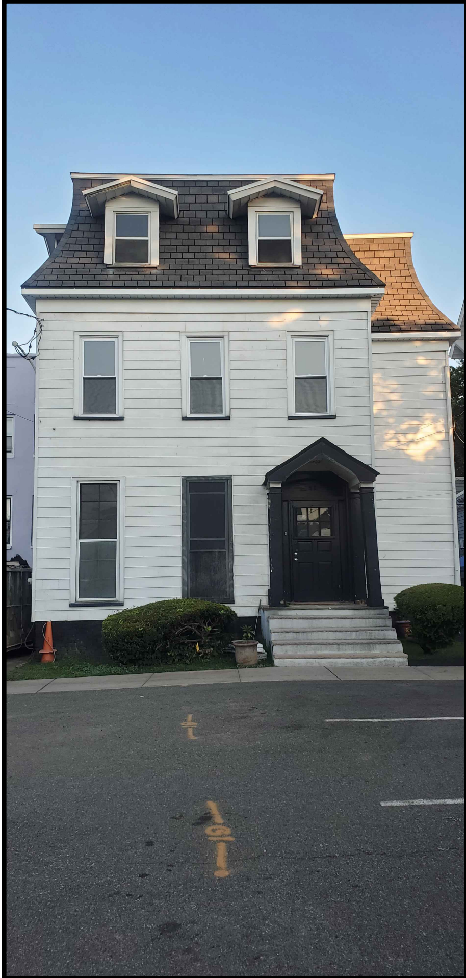
CLOSER VIEW OF FRONT OF BLDG.
