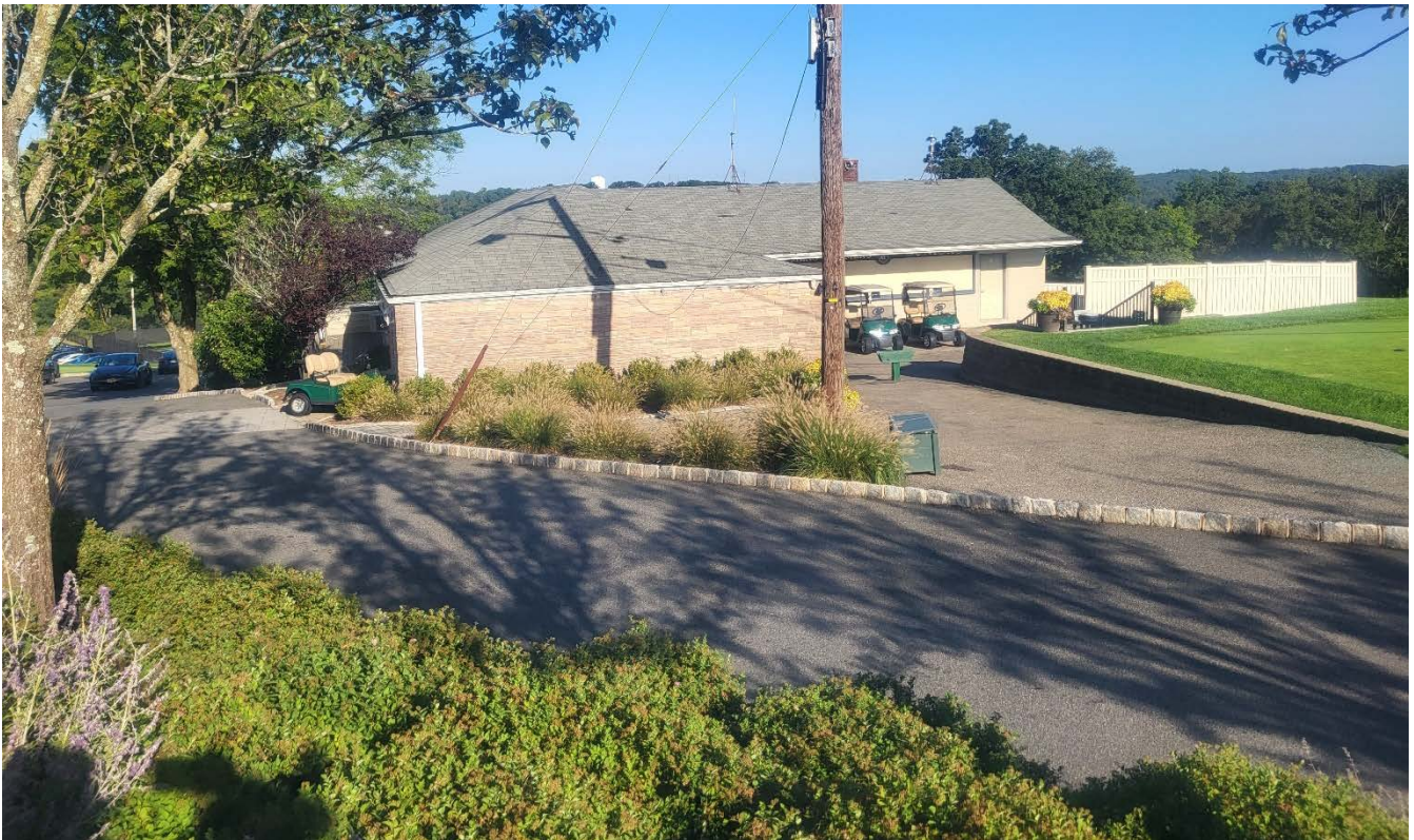
Driveway between upper and lower parking lots and cart barn/pro shop building
