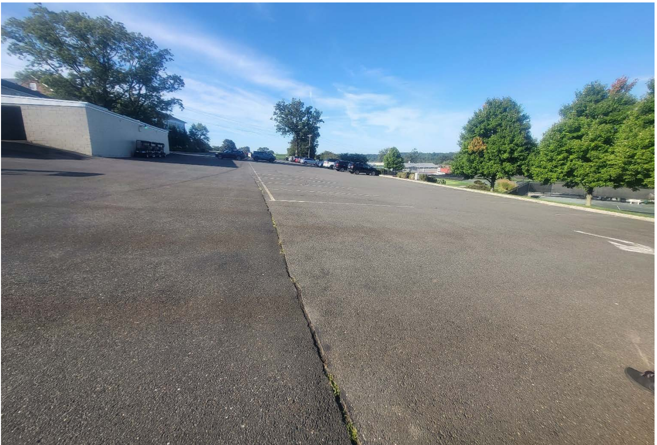
Two views of existing cart barn/pro shop building and parking lot below it
