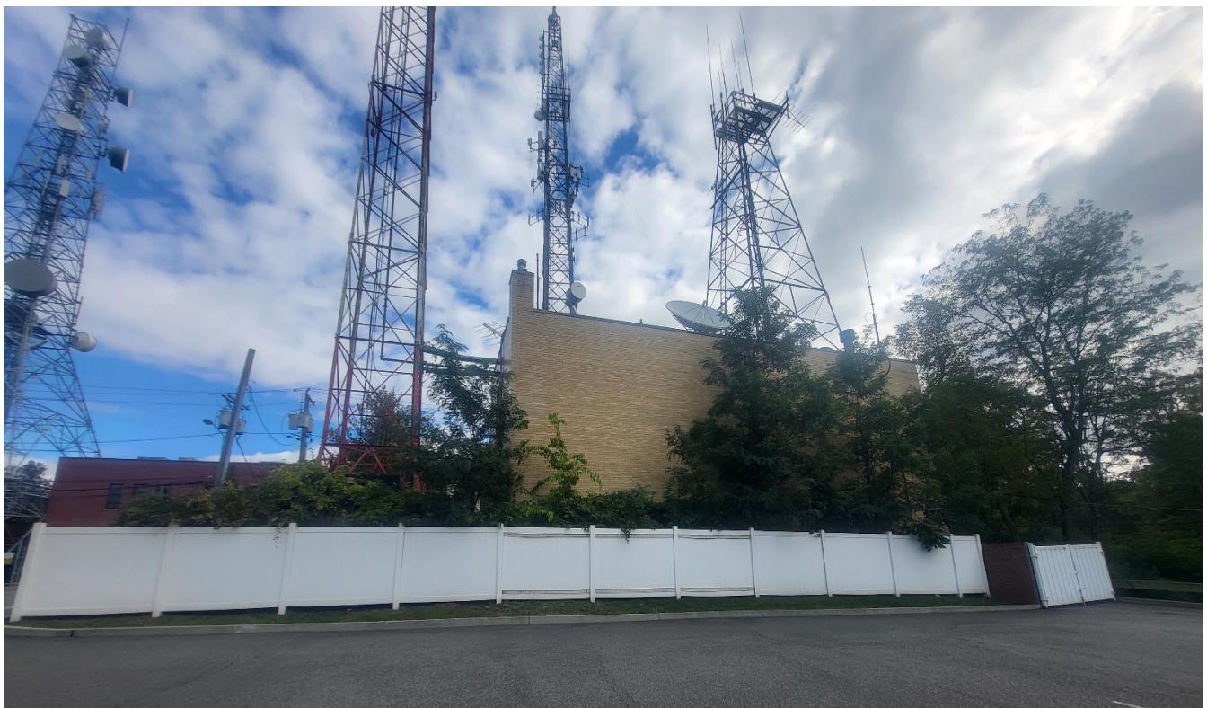
Existing building to be converted viewed from upper parking lot on subject property
