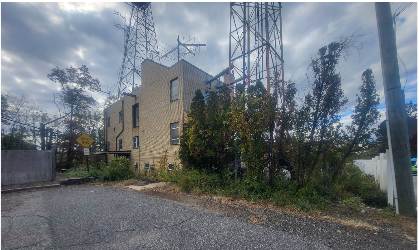
Existing building to be converted viewed from Marcella Avenue
