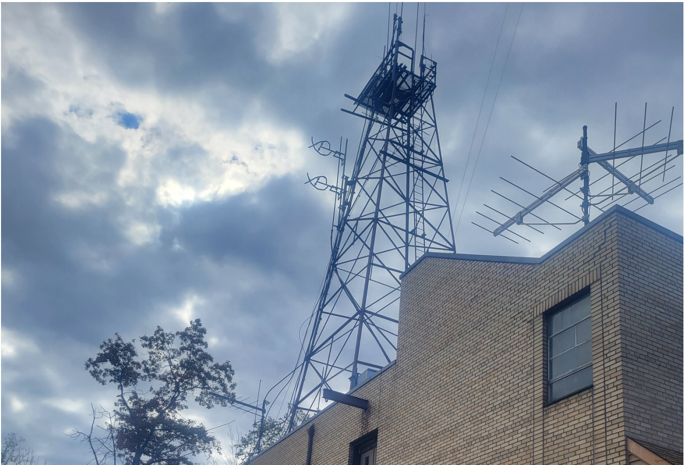
Tower above existing building to be converted
