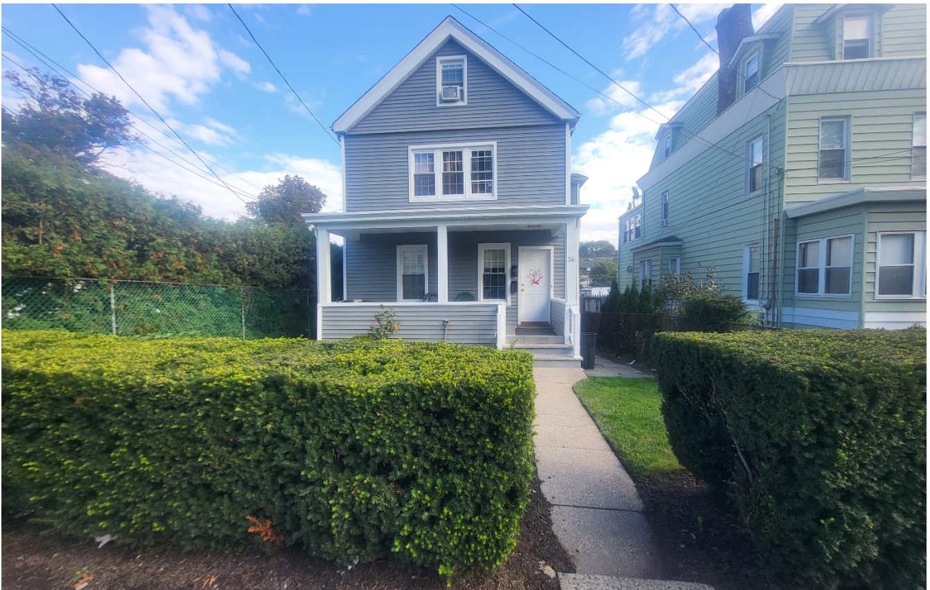
Existing two-family dwelling facing Tompkins Street on proposed Lot A
