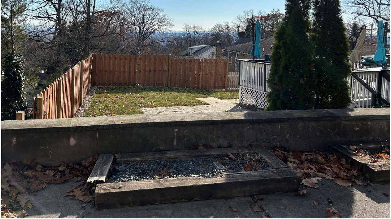
Fence atop rear yard retaining wall
