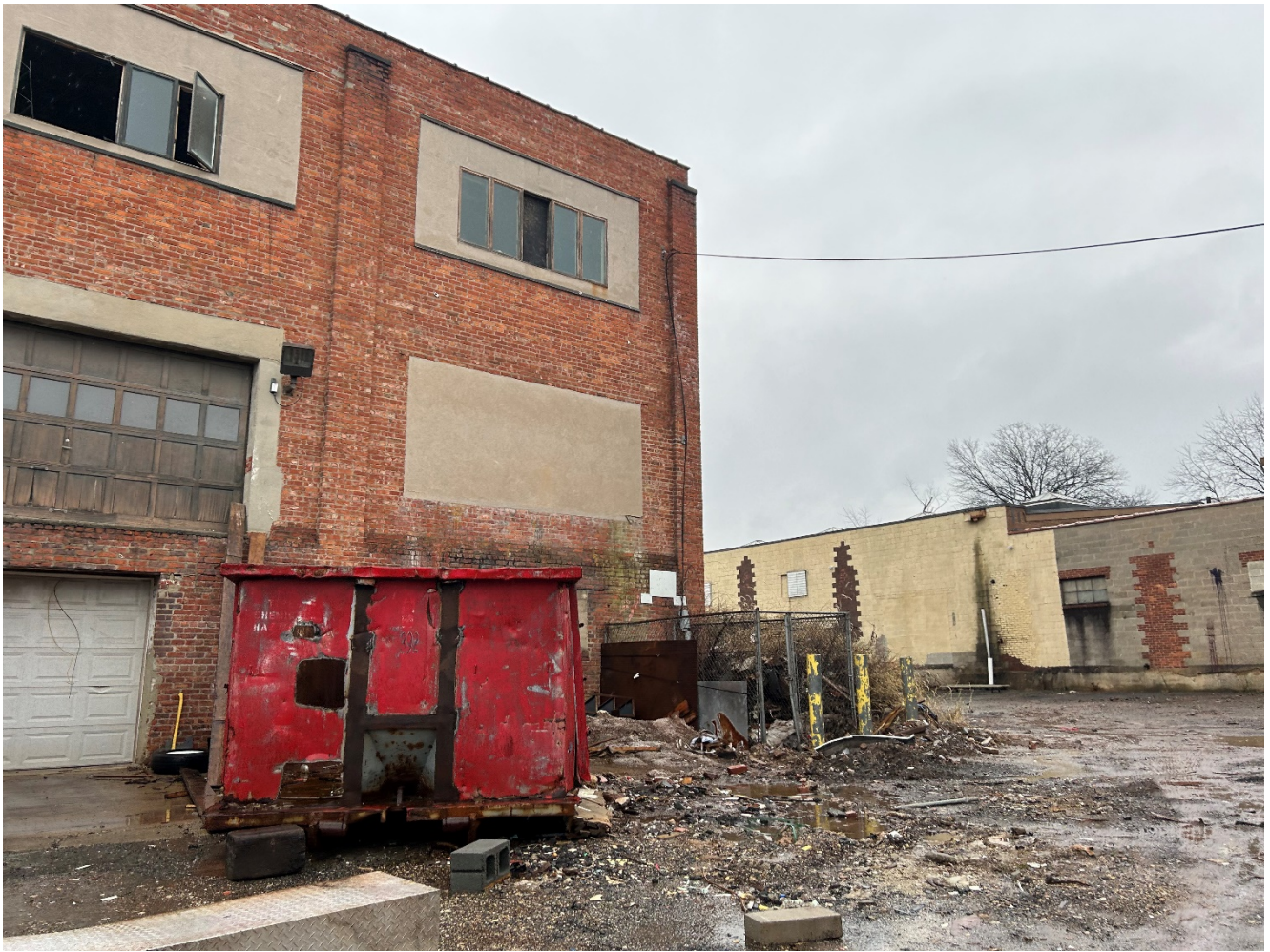
Existing conditions on Lot 22.01
