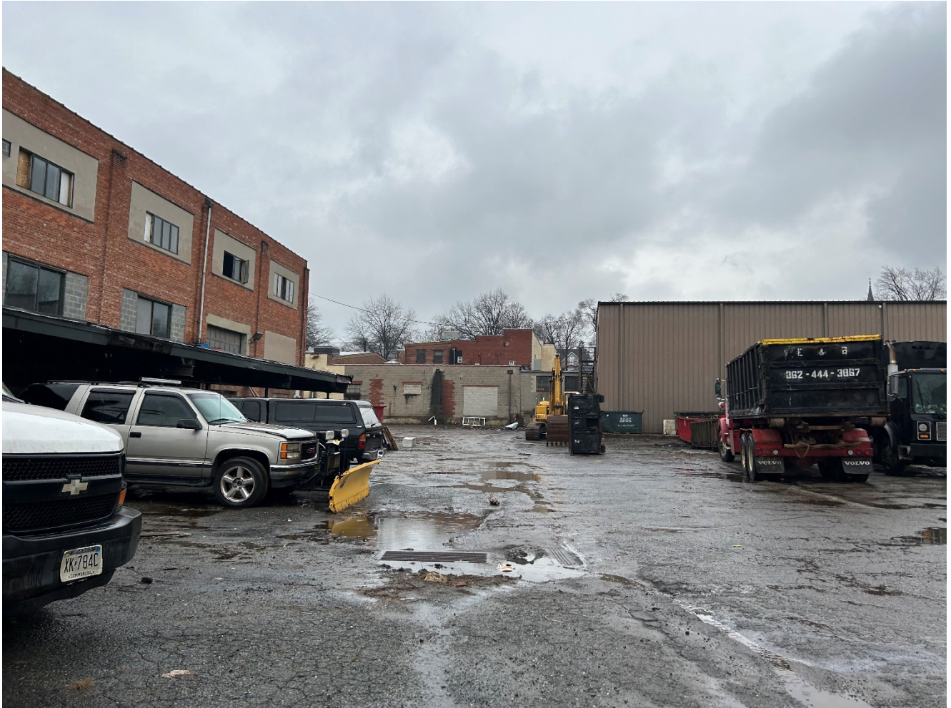
Views of Lot 22.01 looking east from Ashland Avenue
