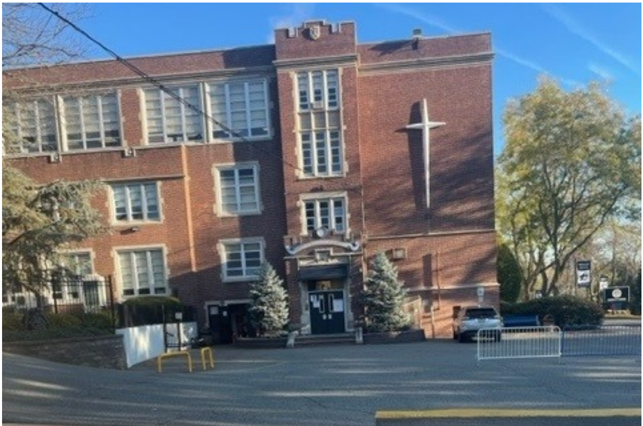
Opposite side of school building from proposed addition
