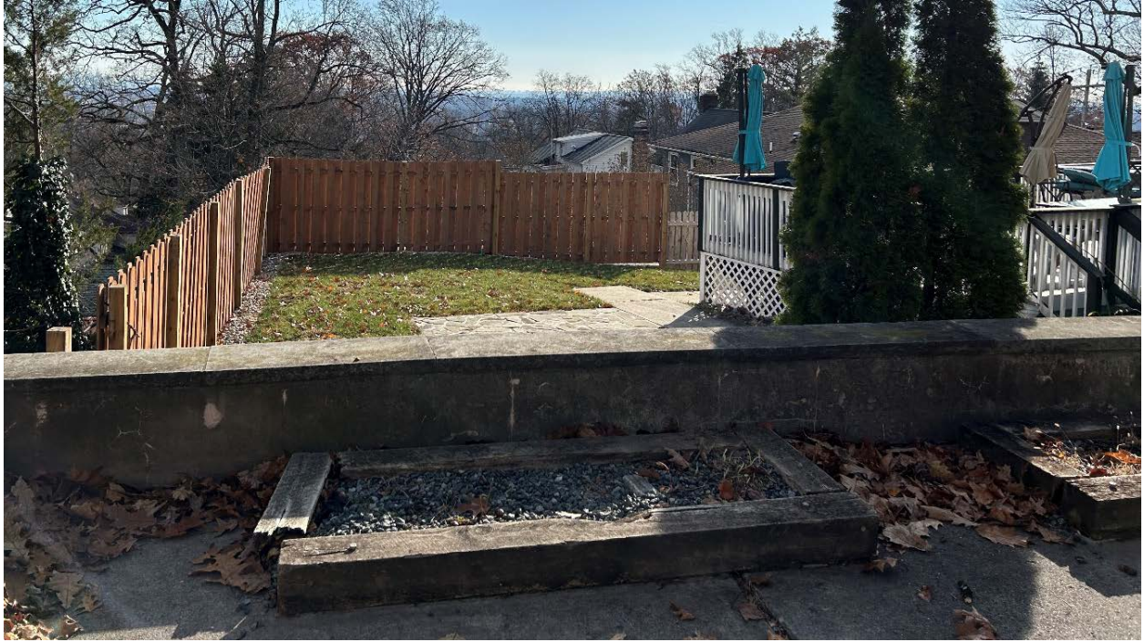
Fence atop rear yard retaining wall
