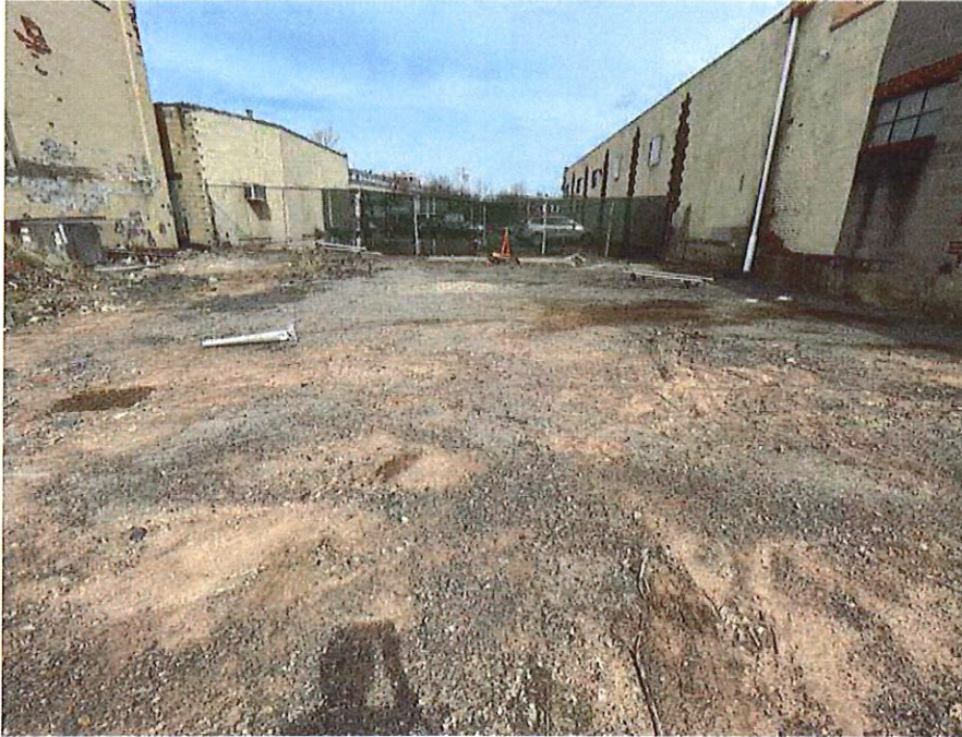
Photo 9: Looking north towards existing parking lot and fence in front of 2-story metal building
