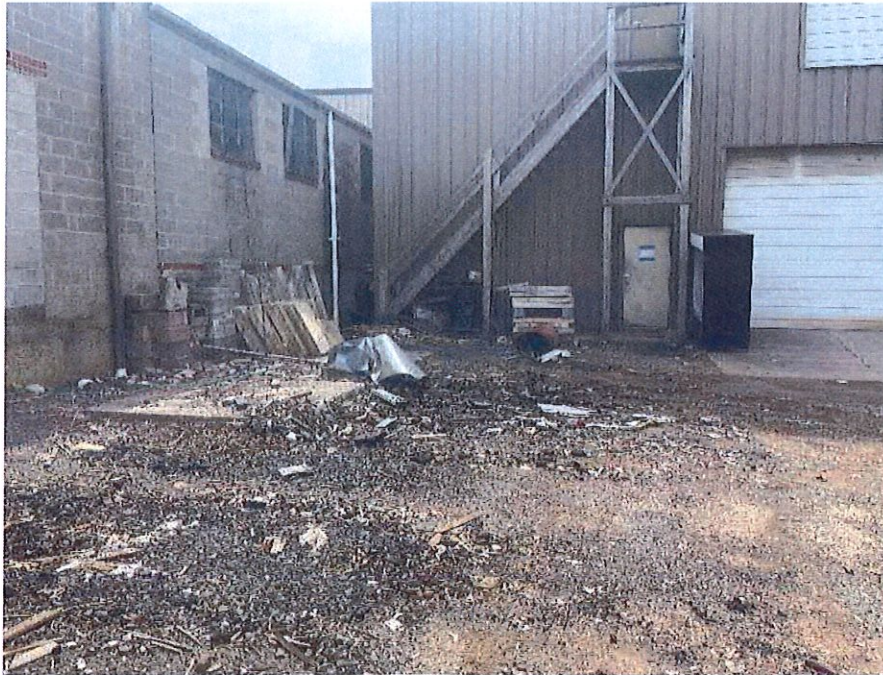
Photo 10: Looking southeast towards existing 2-story metal building
