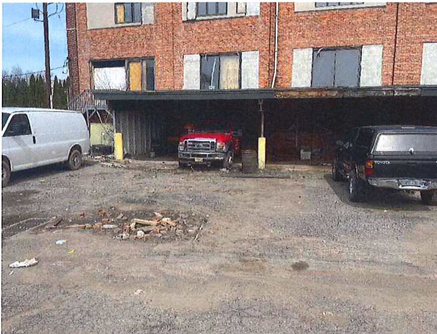
Photo 6: Looking North towards 3-story building
