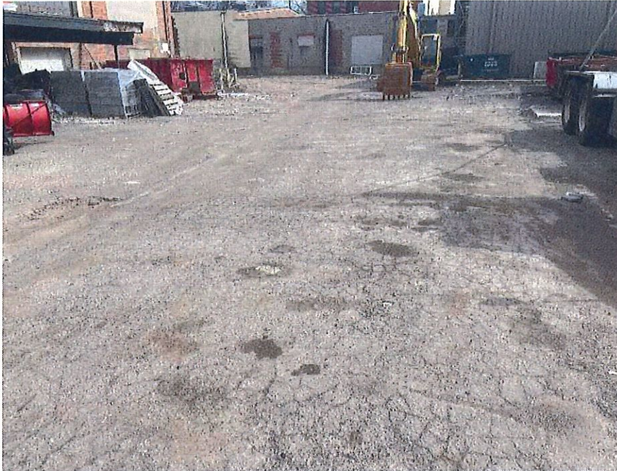
Photo 7: Looking east towards corner of 3-story and 2-story buildings
