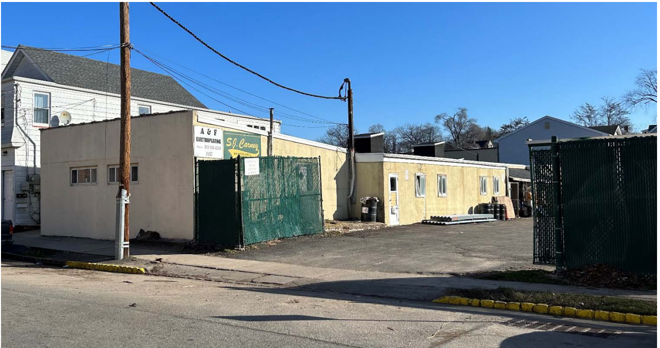
Views along Ashland Avenue frontage
