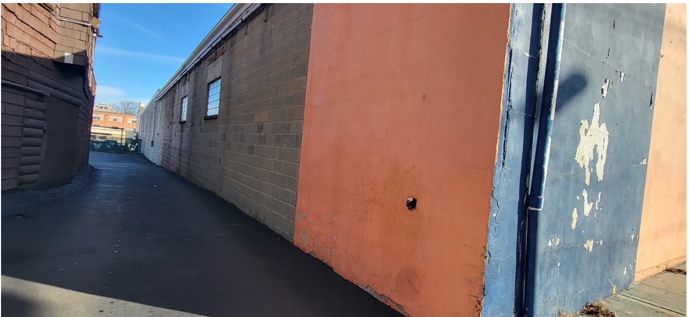
Views along White Street frontage
