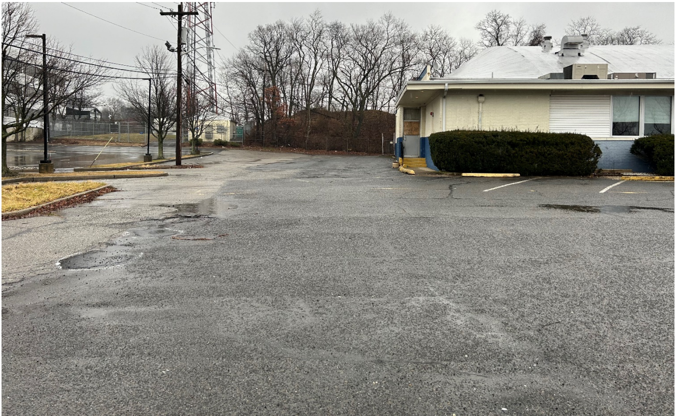
Northwest corner of existing building, with connections to adjacent parking lot on left
