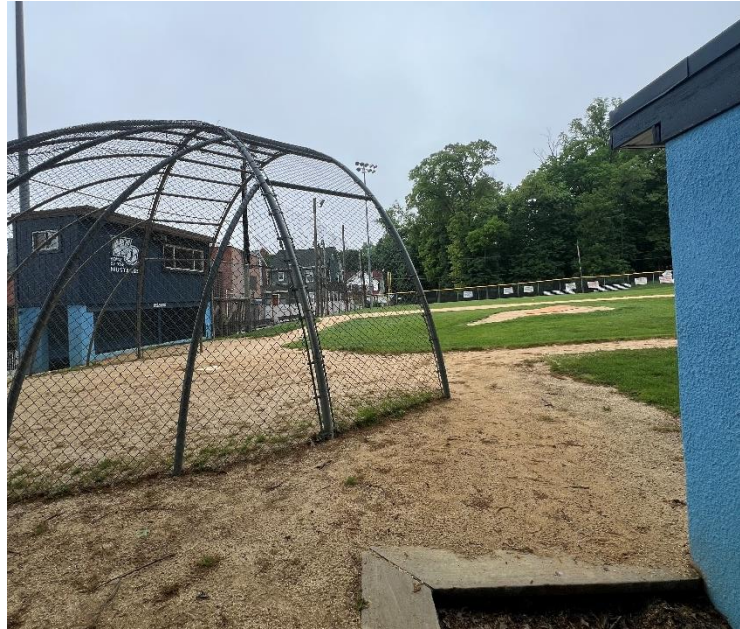
Figure 7: View of existing backstop
