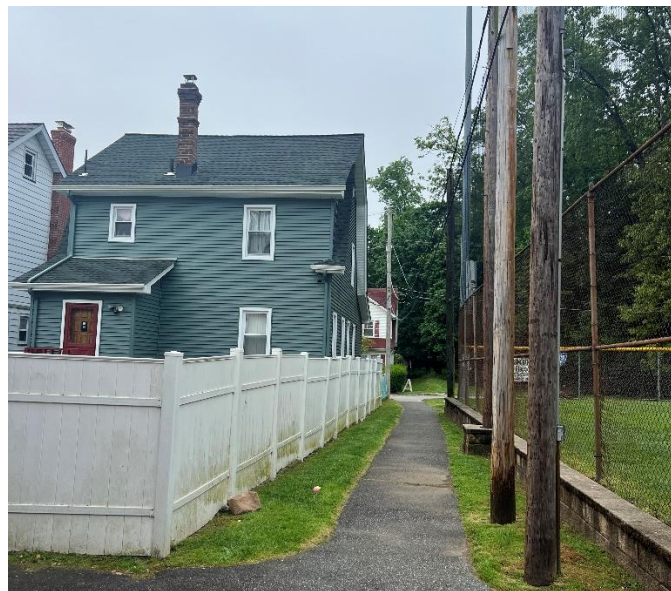
Figure 10: View of third base fence line and buffer to adjacent property to the south
