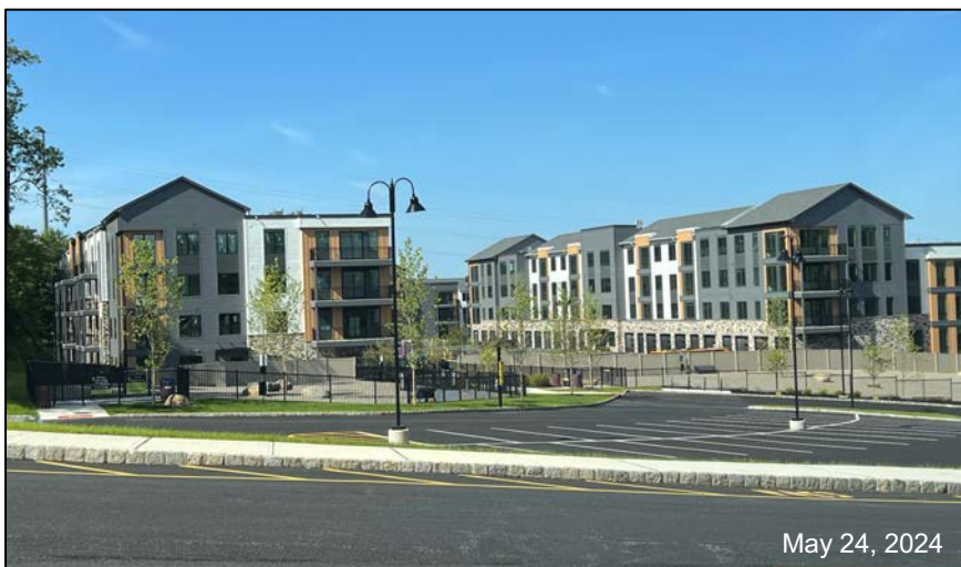
Photo 6: View looking south across the proposed new Lot 42.04 at the residential buildings located on new Lot 42.03.
