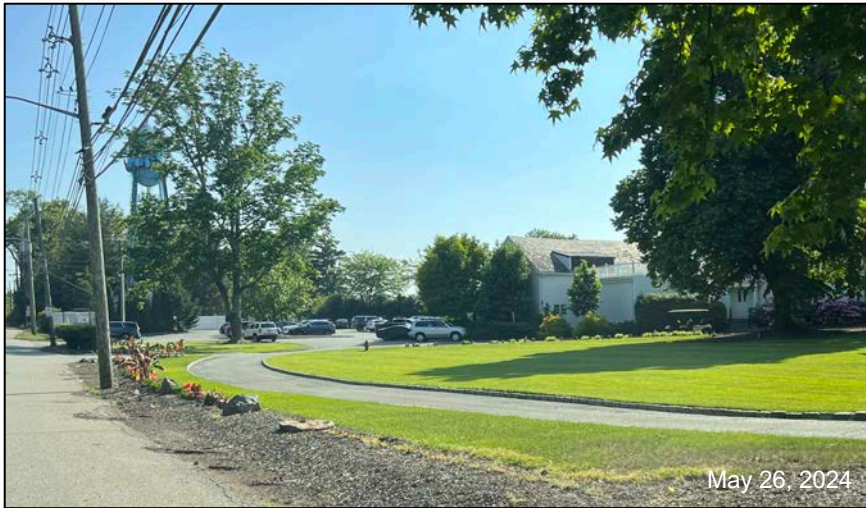
Photo 7: View of the front yard from the north on Prospect Avenue. The applicant proposes to install 15 new parking stalls in this area as well as a new 3-foot-tall wall along the property.
