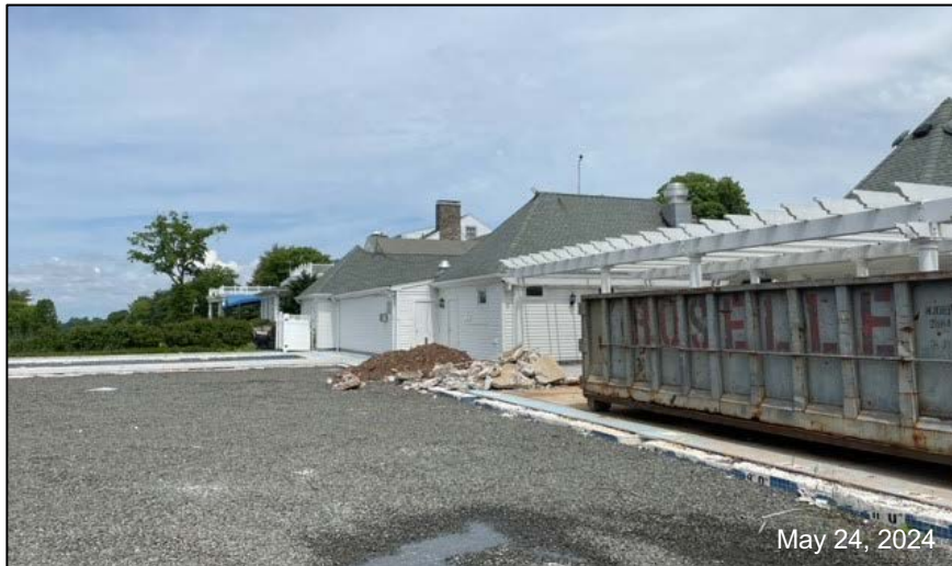
Photo 3: The area on the western side of the existing golf building, where the proposed expansion will be constructed.
