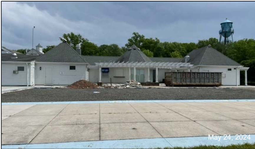
Photo 4: View from the west showing the rear of the existing golf building and the original pool building that will be demolished.
