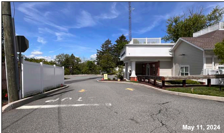
Photo 3: View of the driveway between the existing school building (right) and the location of the proposed annex building (left). A striped crosswalk and signage will be provided here for the safety of children crossing between buildings..
