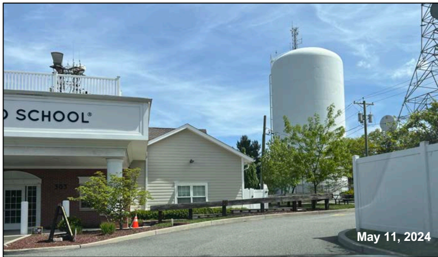
Photo 4: View of the driveway between the two building from the parking area.
