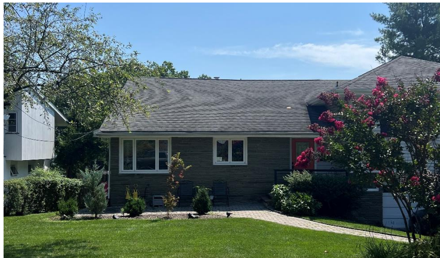
Figure 2: Front yard of 6 Mountain Way South
