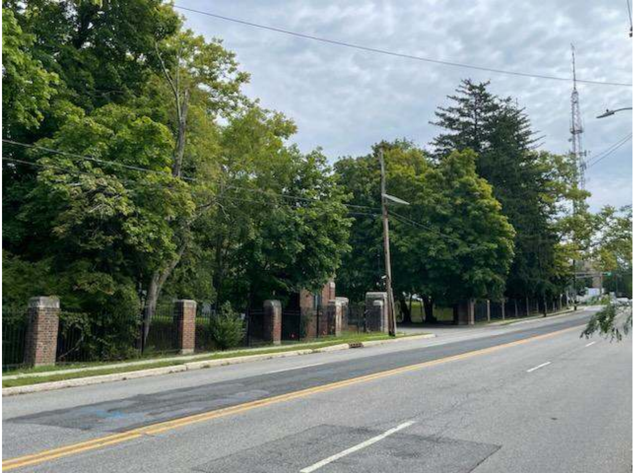
View of fence along Mount Pleasant Avenue, taken August 28, 2024. The entrance to the Station will be reconfigured. Communications/radio facilities are located on the east side of Prospect Avenue.
