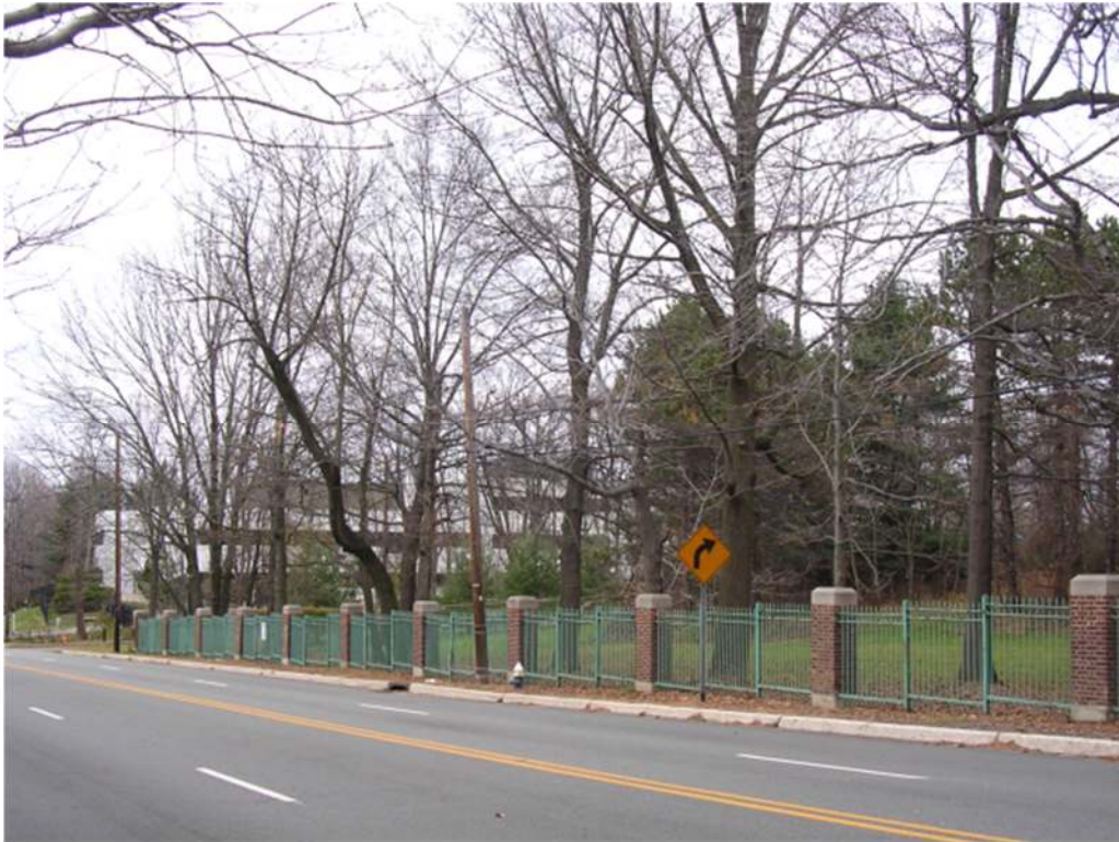
View of fence along Mount Pleasant Avenue in 2007.
