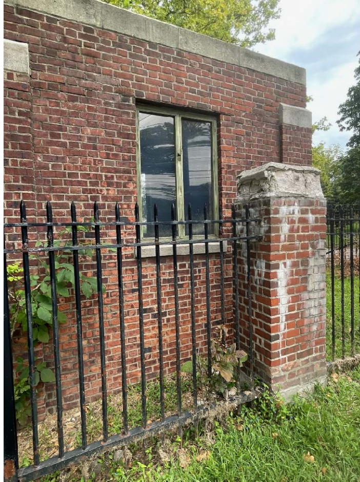
View of station fence and existing guard shack (to be demolished), taken August 28, 2024, showing the condition of existing brick pillars.
