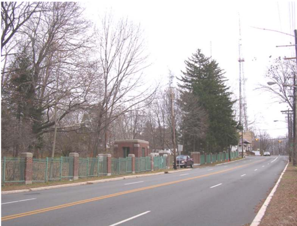
View of fence along Mount Pleasant Avenue in 2007.
