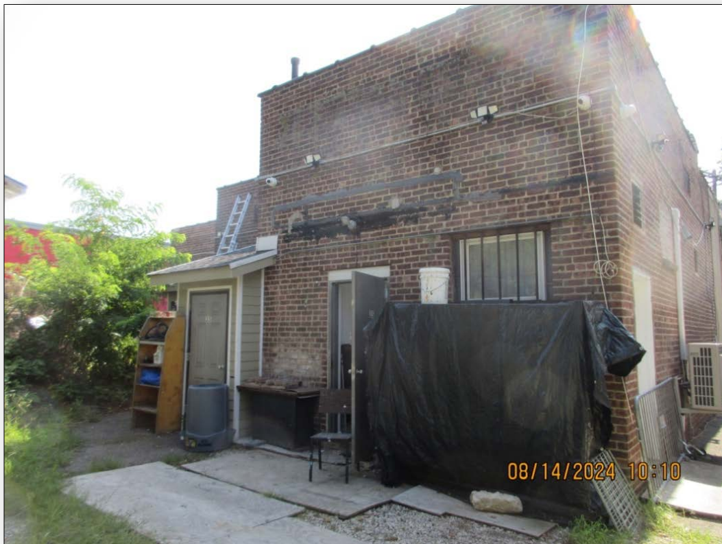
Photo 2: View from southwest showing the rear of the existing building.
