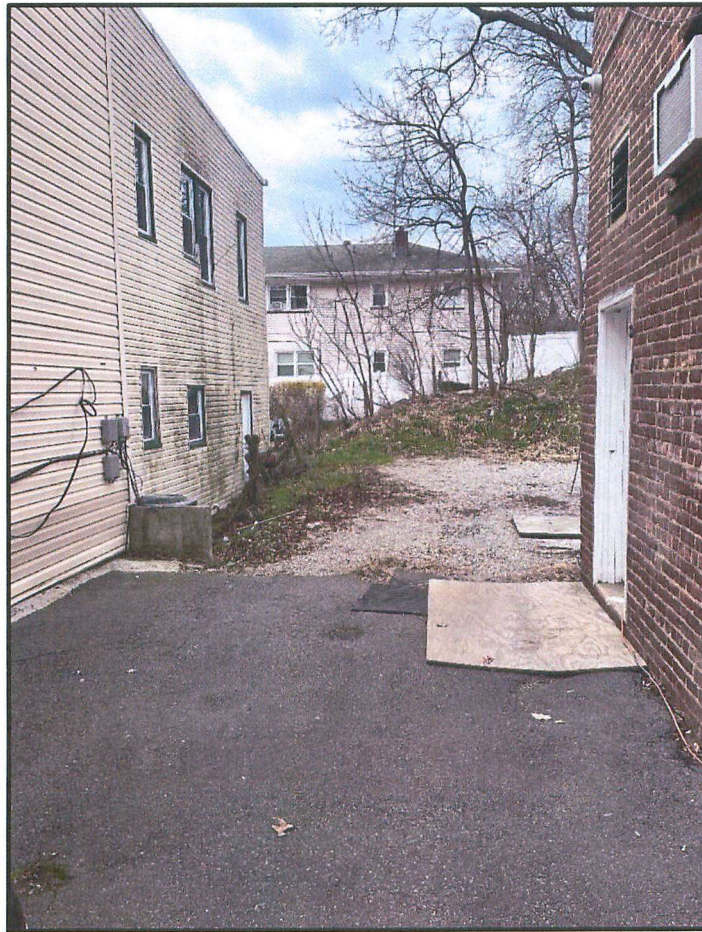
Left Side of Building Viewed from Harrison Avenue
