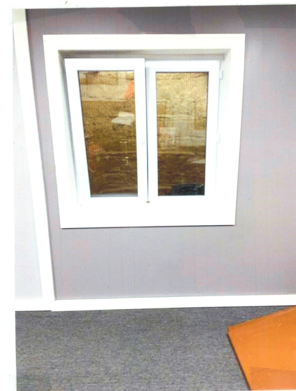
⑤ EMERGENCY ESCAPE WINDOW PHOTOS
