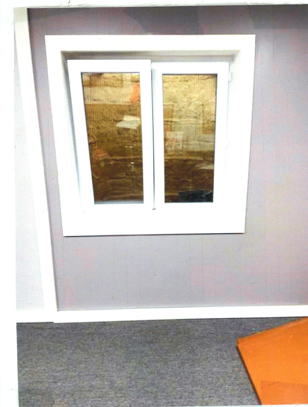
⑤ EMERGENCY ESCAPE WINDOW PHOTOS
