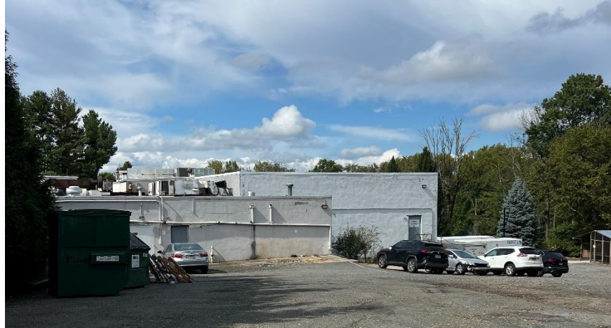
Figure 4: Rear of building used by Wonder Group, Inc. for food preparation
