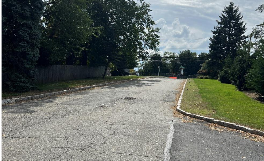
Figure 2: Entrance to site from Eagle Rock Avenue
