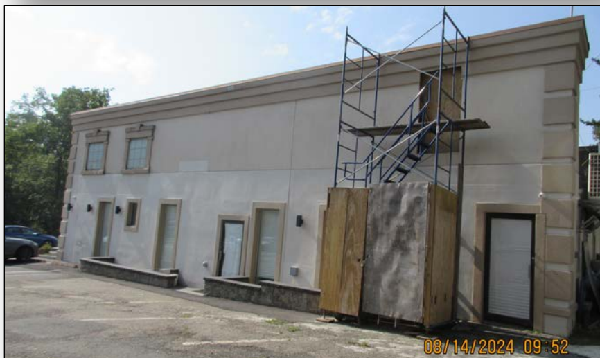
Photo 3: View of the northern side frontage.
