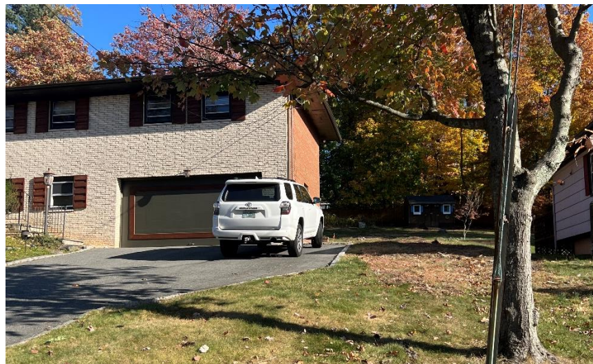
Figure 3: Southern side yard view of 15 Edgewood Ave North where two-story addition is to be located. Note existing roof overhang.
