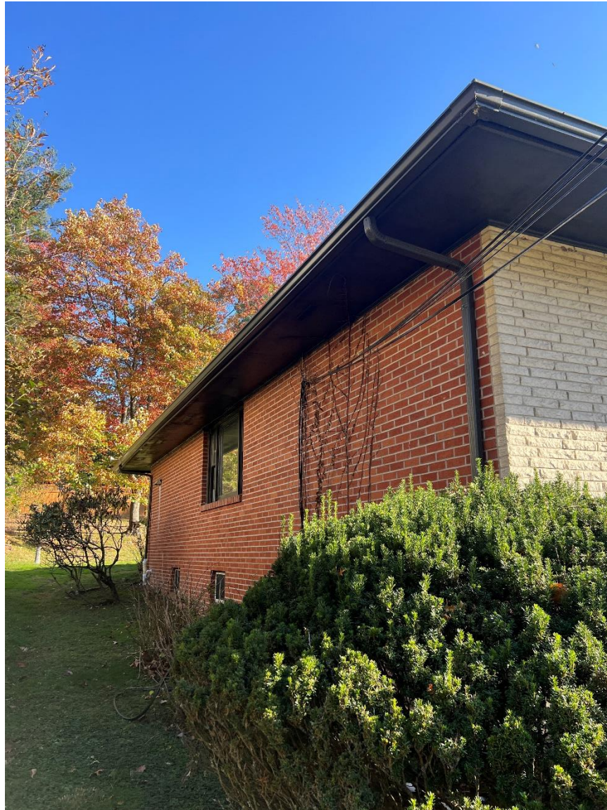
Figure 4: Northern side yard view of 15 Edgewood Ave North where heat pump and emergency escape window are to be located. Not existing roof overhang.
