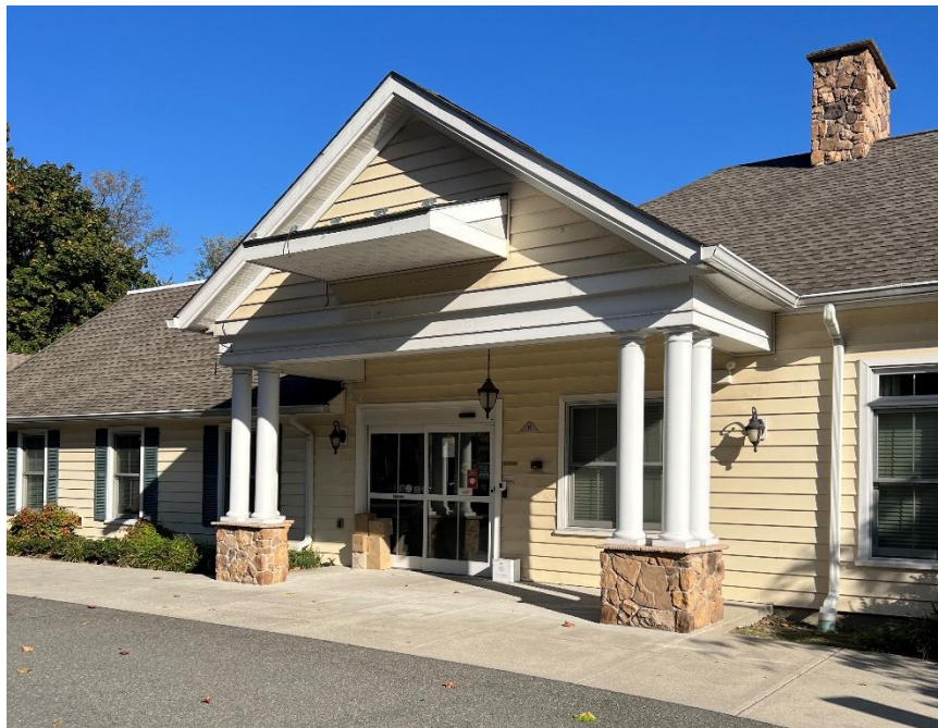
Figure 5: Side entrance at rear building
