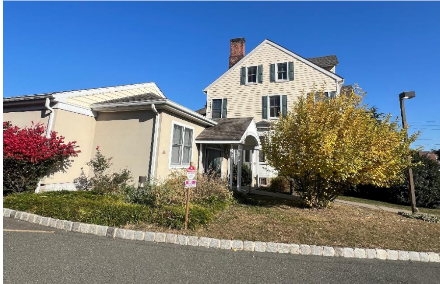
Figure 4: Side of Building
