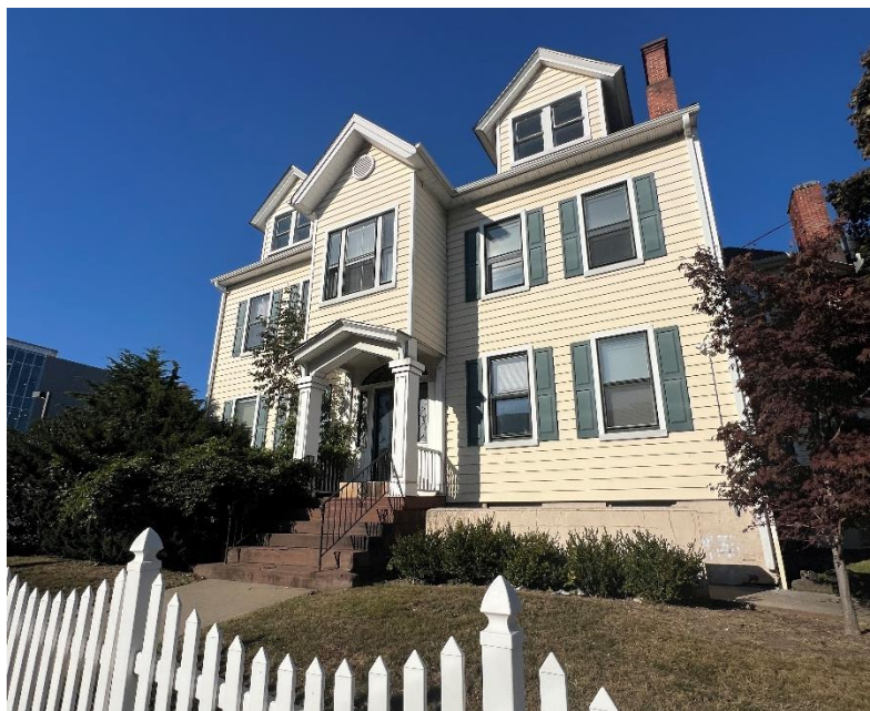
Figure 3: Front of Building
