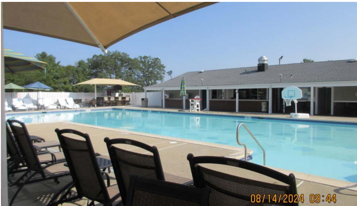
Photo 5: View from the south showing the rear of the existing pool house building that will be renovated and the pool along with the existing canopies.
