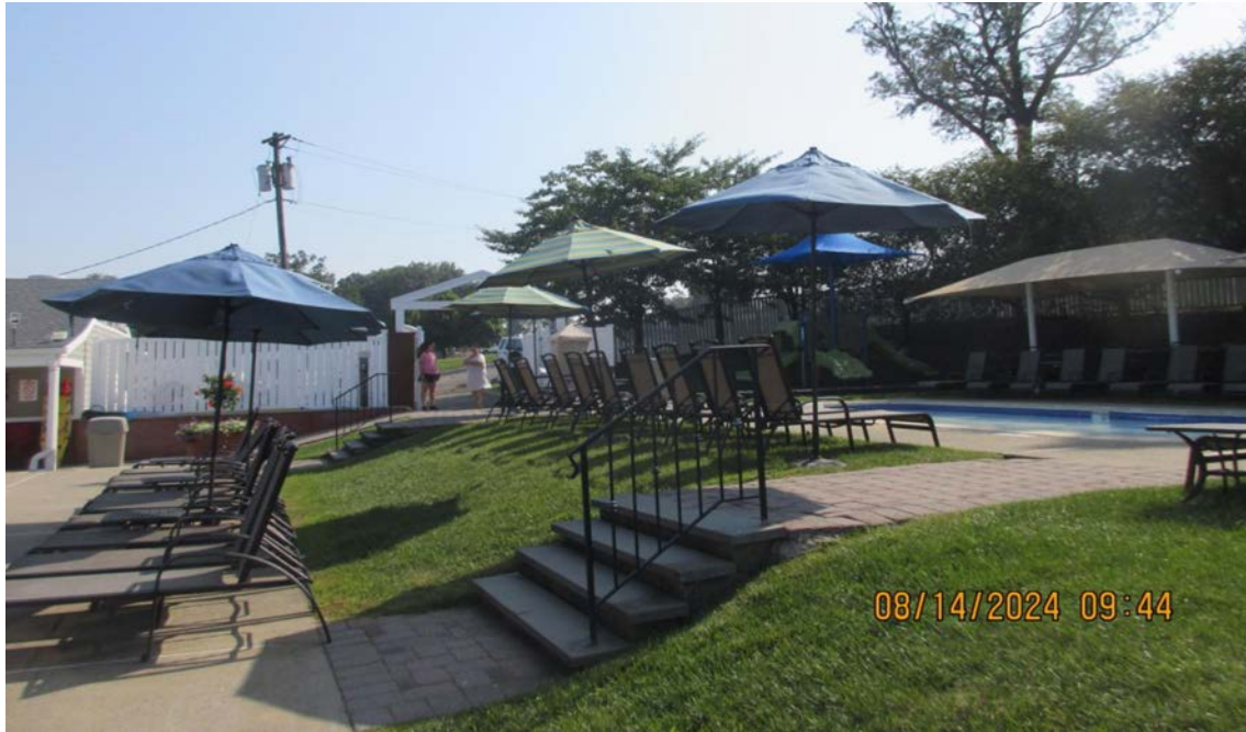
Photo 4: View from the south showing the smaller inground pool and the existing staircase where a new ADA ramp will be installed.
