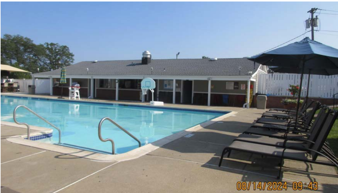
Photo 3: View from the south showing the rear of the existing pool house building that will be renovated and the pool.
