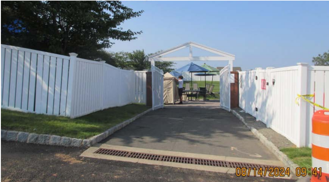
Photo 2: View from the north showing the entrance to the pool area. It is situated between the inground pools.
