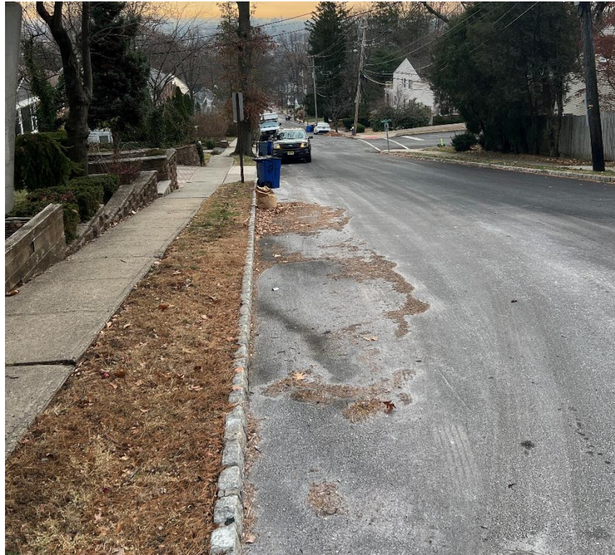
Figure 6: Bradford Ave topographic change looking away from Northfield Ave
