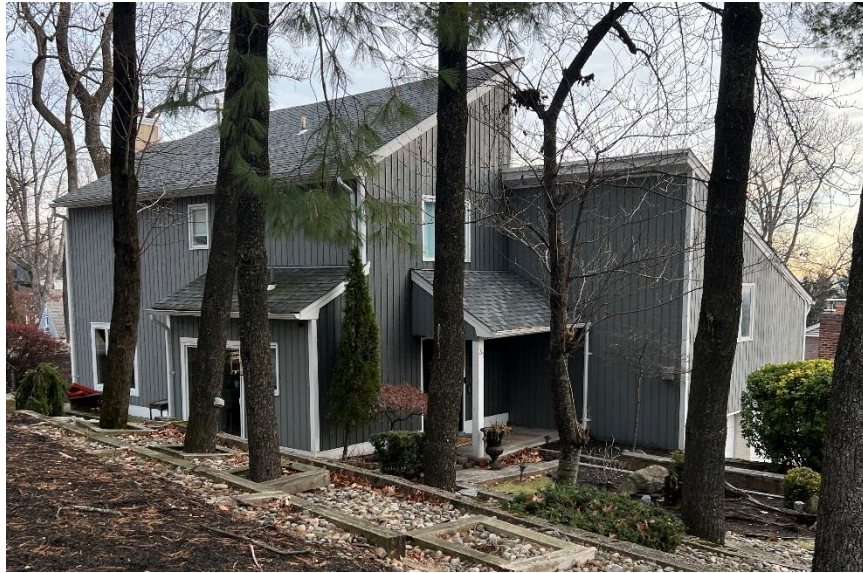
Figure 4: View of property from Northfield Ave
