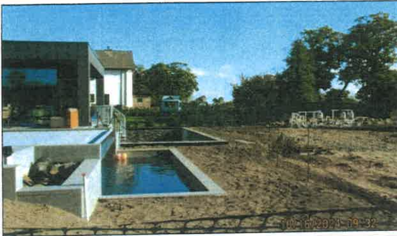
Photo 4: View of the area on the northern side of the pool and pool house.
