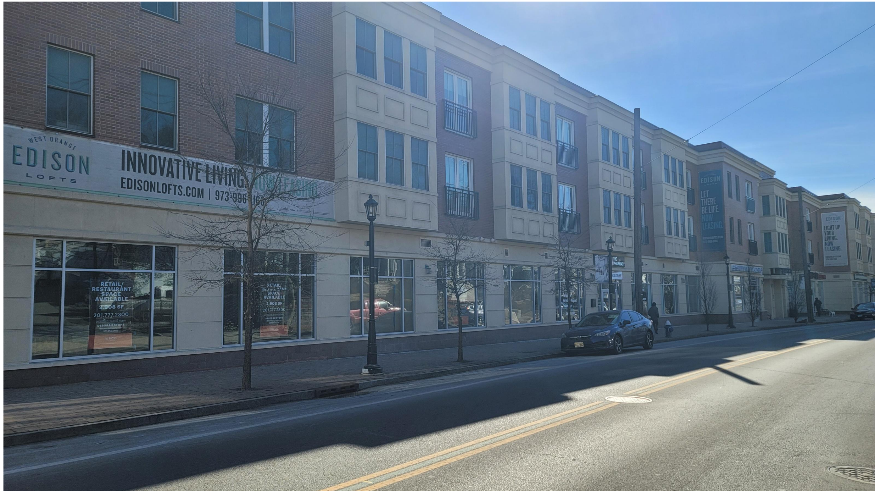
STREET VIEW OF EDISON LOFTS ACROSS MAIN STREET FROM SUBJECT SITE (TAKEN BY JOHN MCDONOUGH ASSOCIATES ON FEBRUARY 5, 2025)
