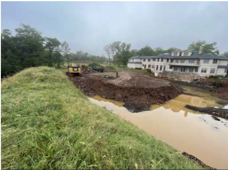
Fig. 1. Temporary berm preventing stormwater from flowing down the mountain.
