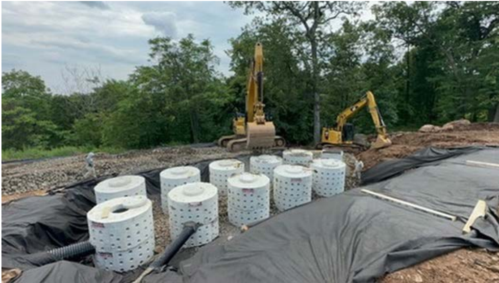
Fig. 2. Installation of 10 (double height) seepage tanks.
