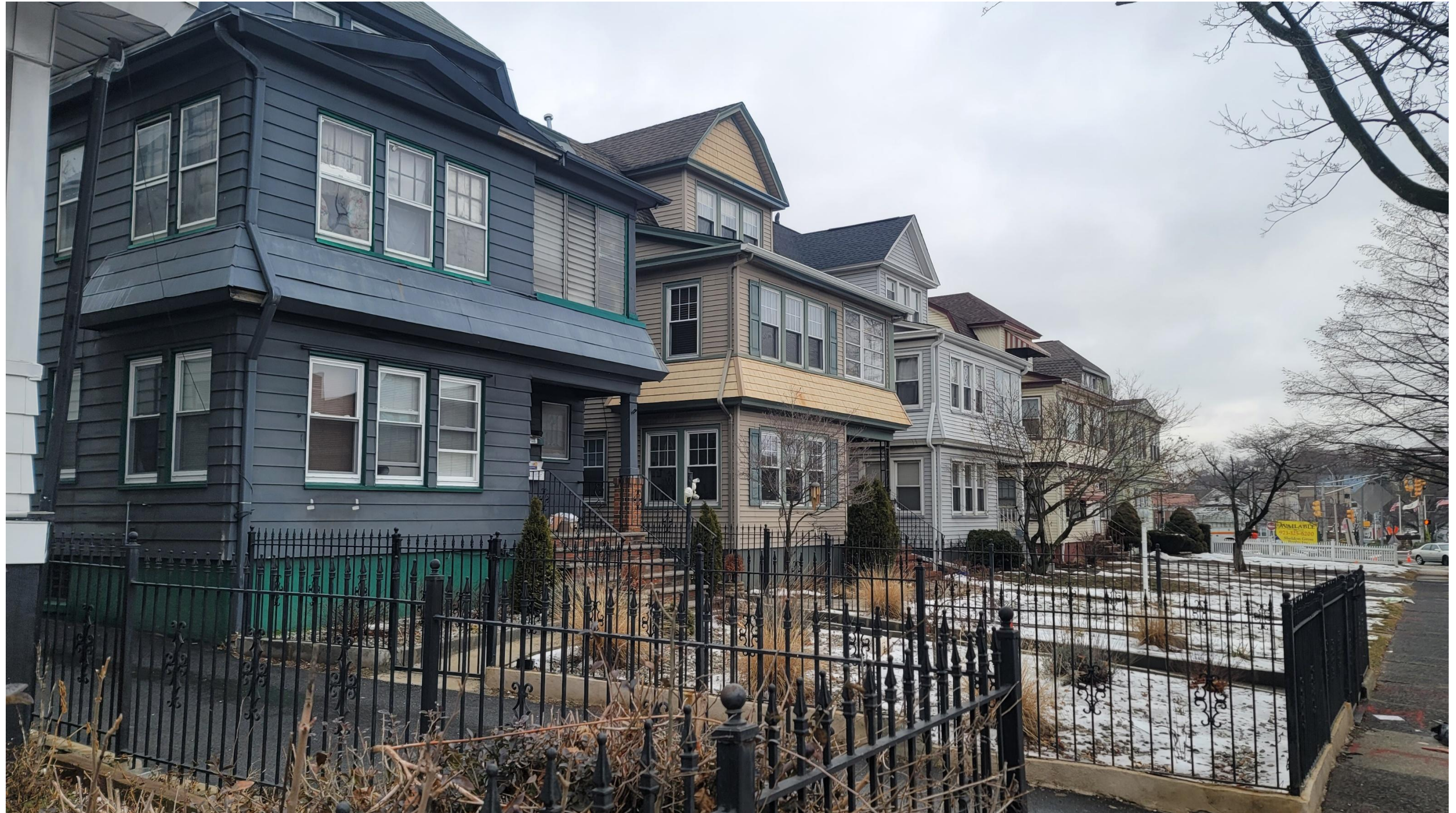
VIEW OF NEIGHBORING BUILDINGS MOUNT PLEASANT AVENUE (TAKEN BY JOHN MCDONOUGH ON FEBRUARY 13, 2025)
